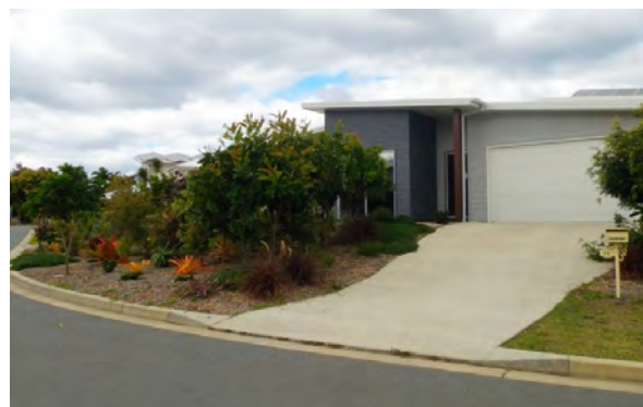
No pedestrian access along verge. Keep mulch away from gutter.
