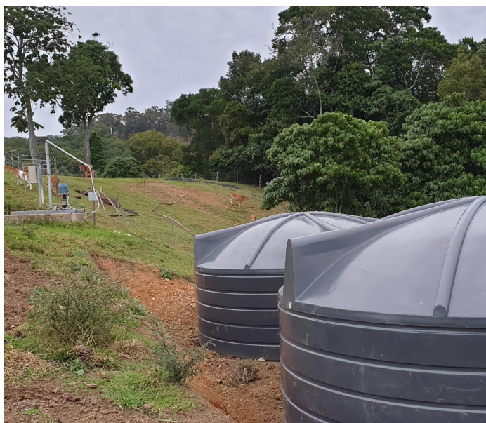
Additional waste water storage tanks installed as part of the project.
