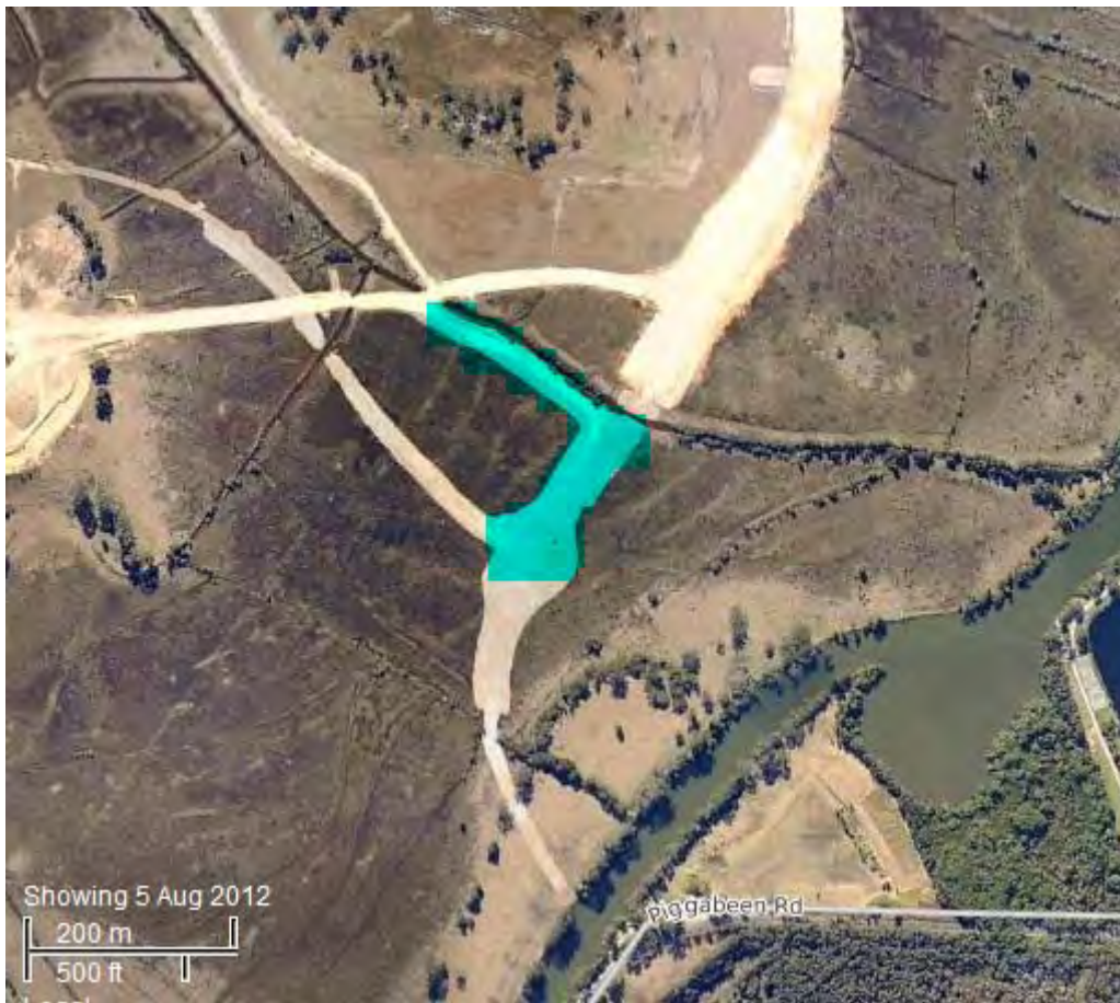
FIGURE 5 – BLUE HIGHLIGHT INDICATES WORKS IDENTIFIED ON SITE ON 3 JULY 2012
