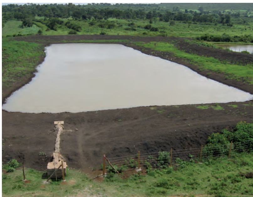
The heart of Gona Dam now - filled with usable water after Safewater 4.
