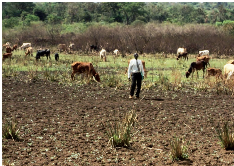
The area where Gona Dam now stands in March 2011 prior to earthworks.
