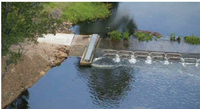
Bray Park Weir
