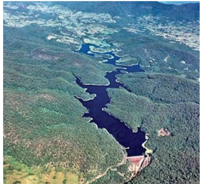
Clarrie Hall Dam
