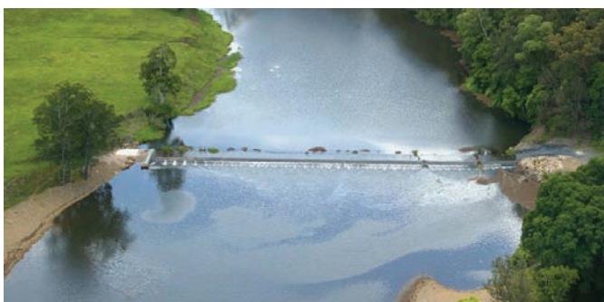
Bray Park Weir
