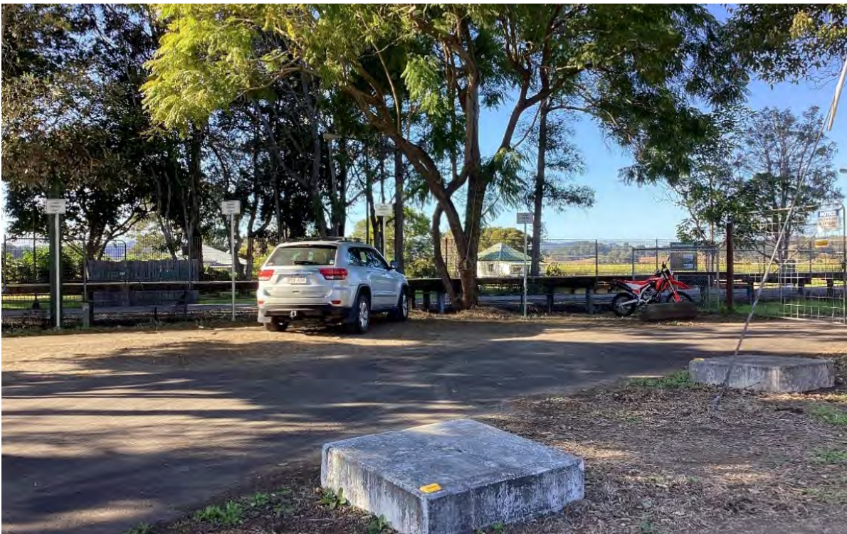
Picture 38 Proposed cut location from the east
