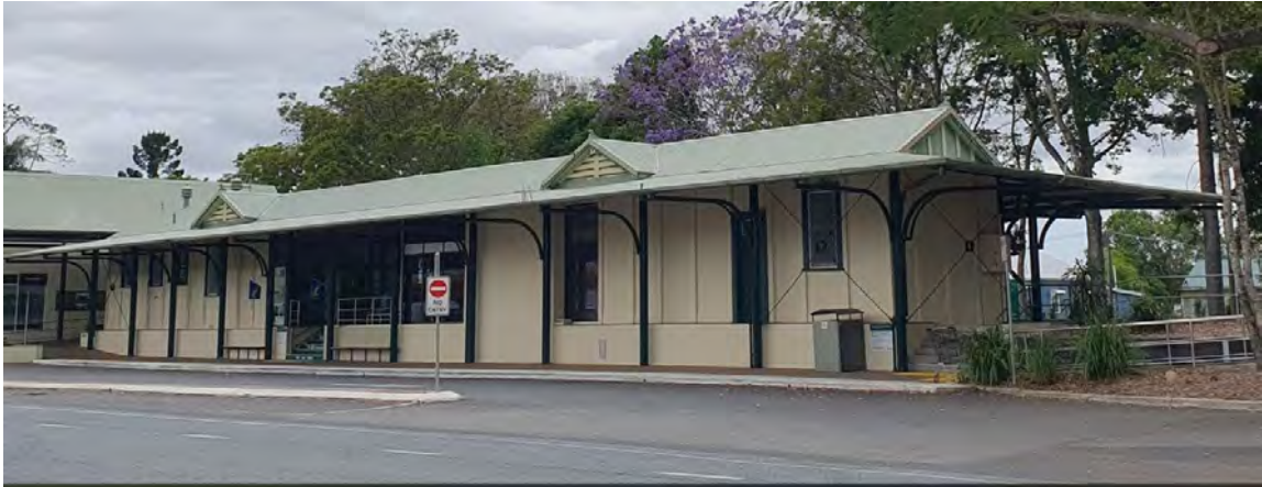
Picture 6 Western elevation of 1920s building
