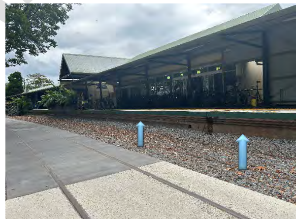
Picture 28 Proposed location for two directional signs below platform (Signage 5)
