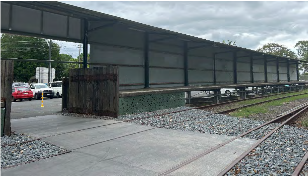
Picture 41 Ground surface treatment of northern access point
