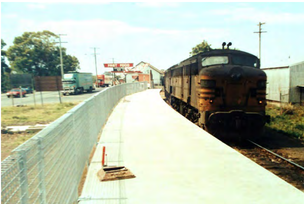
Picture 5 – Extended Platform, 1985 Source: NSW Railways Past and Present
