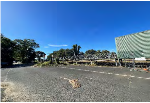
Picture 23 Fencing viewed from carpark and facing Tweed Valley Way
