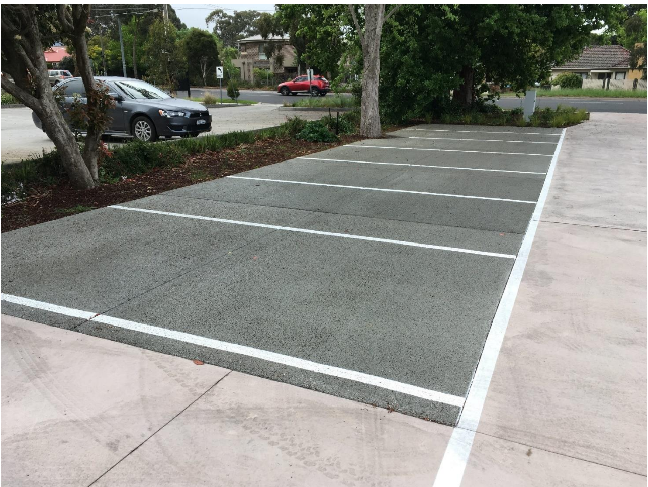
Figure C1: WaterPave carpark in structural root zone and tree protection zone of tree
