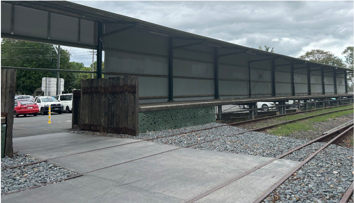
Picture 5 Ground surface treatment of northern access point
