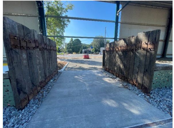
Picture 4 Existing sleepers at northern entrance
