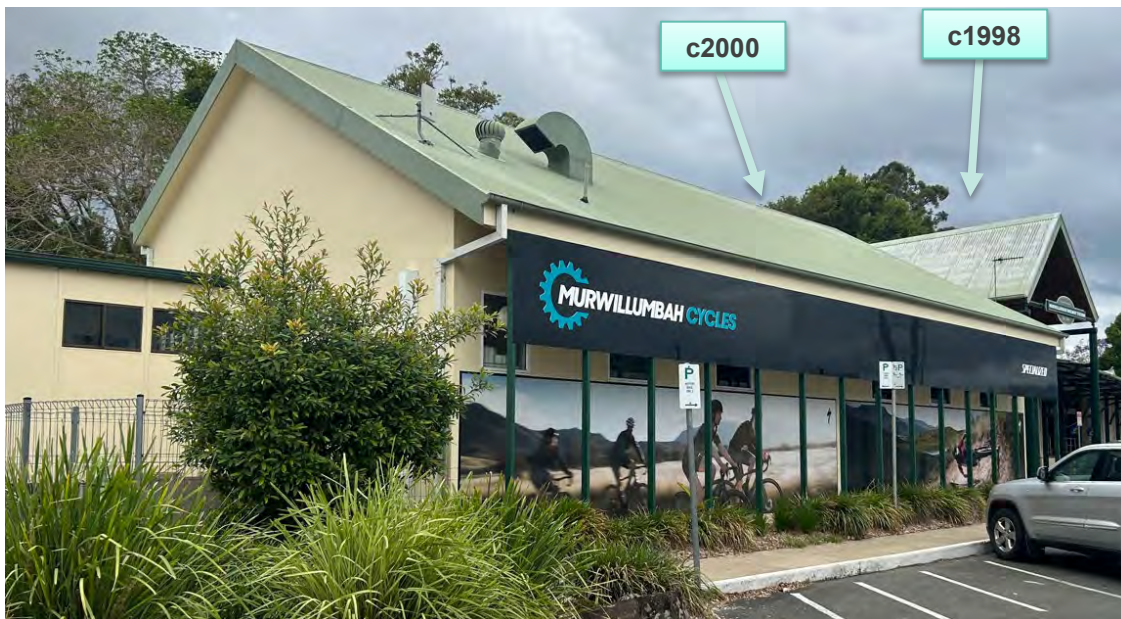
Picture 14 Western elevation of 1990s and 2000s roofs (Picture 14)
