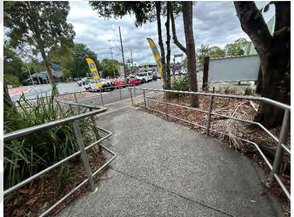
Picture 12 The existing northern access ramp to the platform
