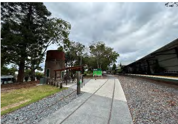
Picture 15 Existing staging area
