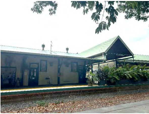
Picture 21 Proposed location on 1920s station building
