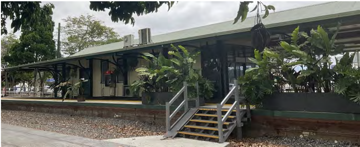
Picture 7 Eastern elevation of 1920s building
