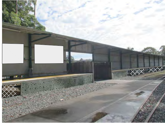
⑦ Screens or signage to be hooked to the side of the platform
