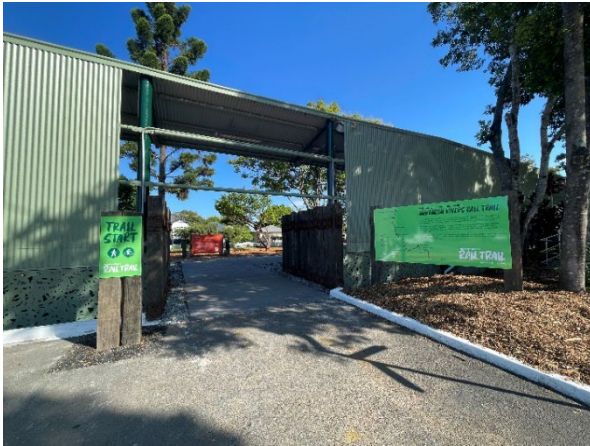
Picture 3 Existing sleepers at northern entrance
