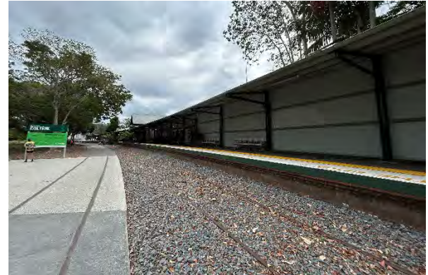
Picture 14 Location of proposed staging area extension from north
