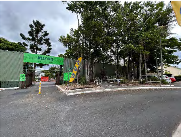
Picture 11 Existing non-compliant ramp viewed from the carpark
