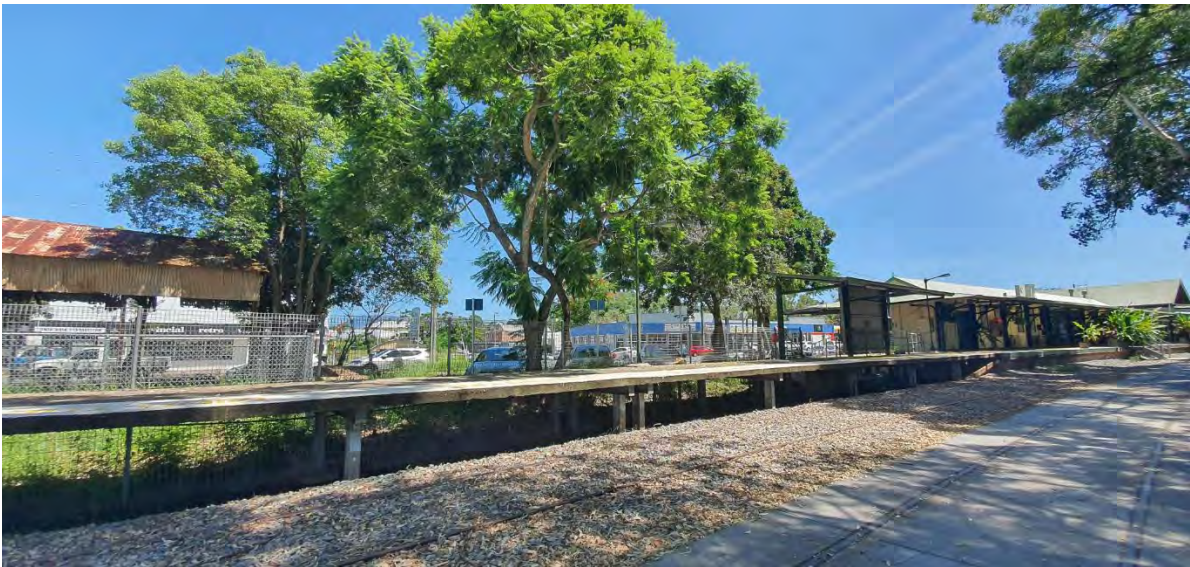
Picture 37 Proposed cut location from the east
