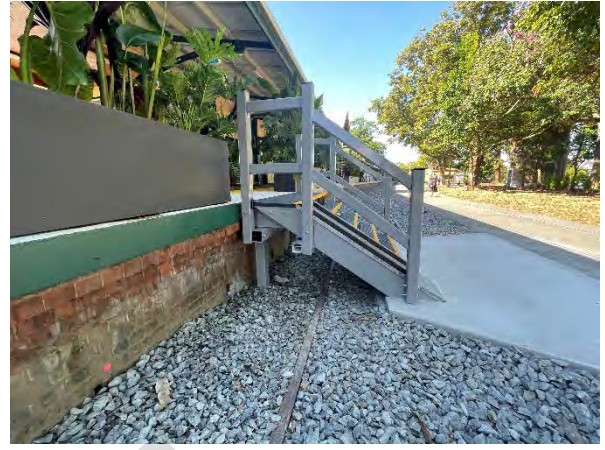
Picture 10 Stair abutting platform
