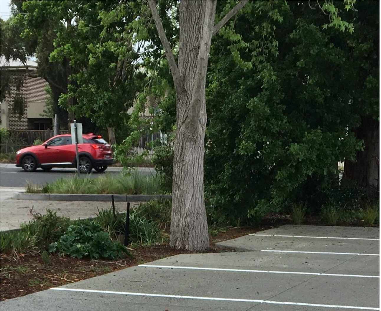
Figure C2: Zoomed in photo of above photo showing WaterPave carpark in structural root zone and tree protection zone of tree
