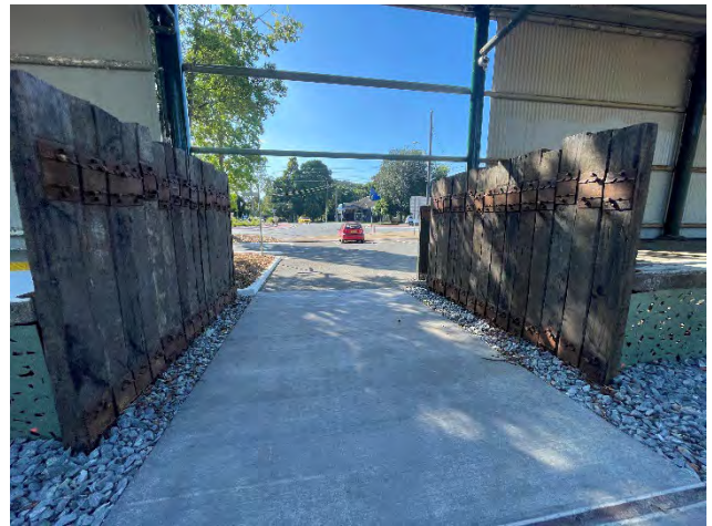
Picture 40 Existing sleepers at northern entrance
