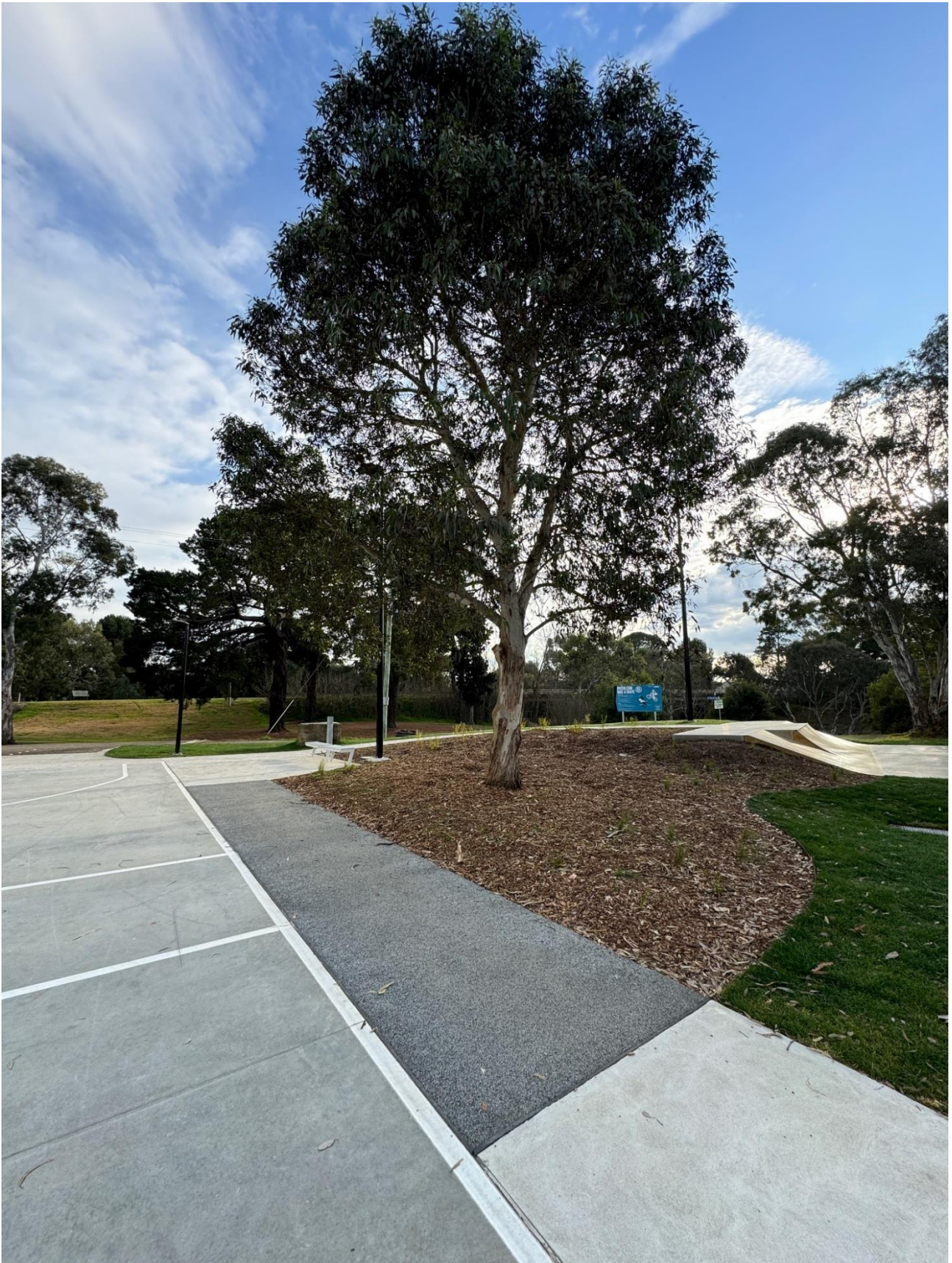
Figure C4: WaterPave section of footpath between garden bed and concrete carpark, within structural root zone and tree protection zone of tree
