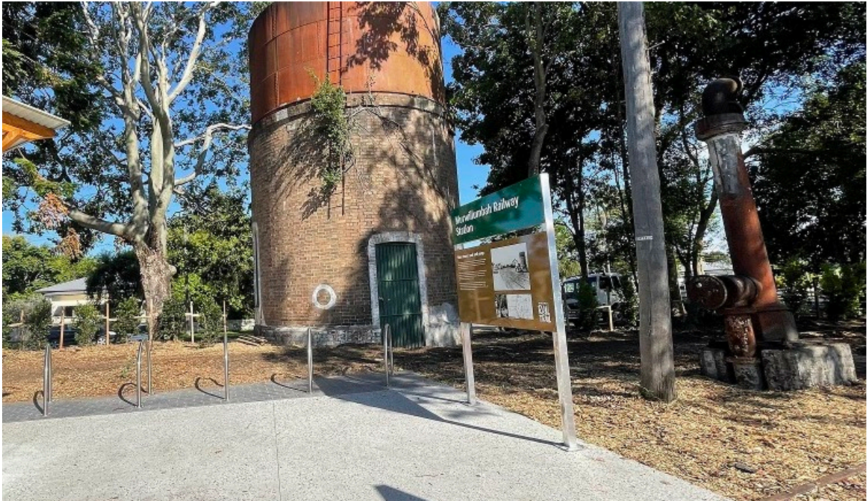
Picture 12 Existing bike racks at northern end of Murwillumbah Railway Station Complex
