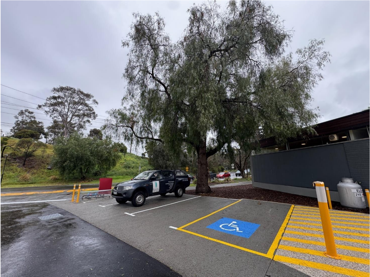
Figure C3: WaterPave accessible carpark in structural root zone and tree protection zone of tree
