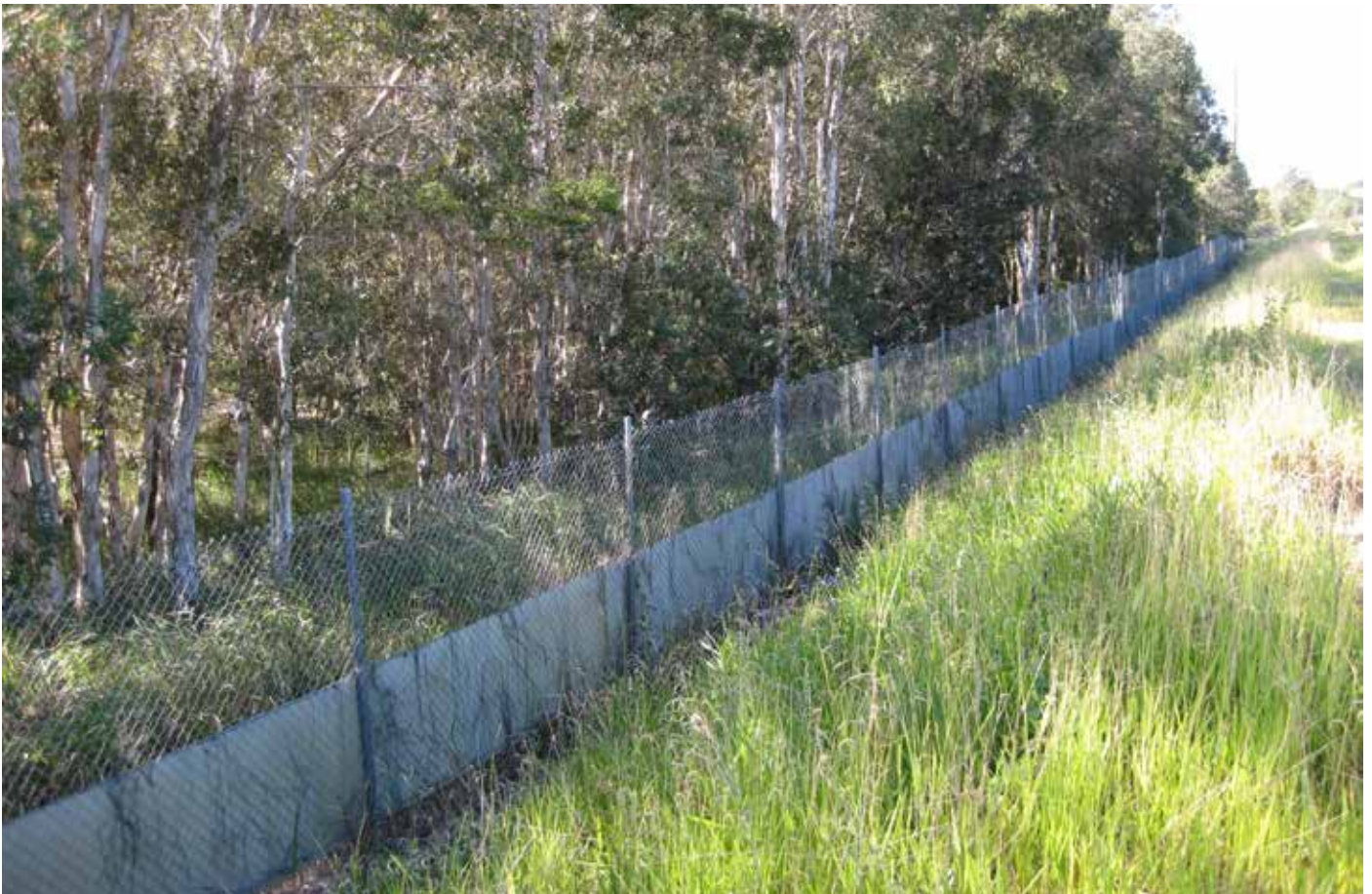
Wildlife exclusion fencing along Tweed Coast Road helps prevent wildlife such as koalas, wallabies and bandicoots from accessing busy roads where they are vulnerable to motor vehicle road strike.
