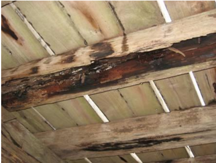
Figure 7 - Example Timber Bridge Super Structure (Bridge Girder) Condition Score 5
