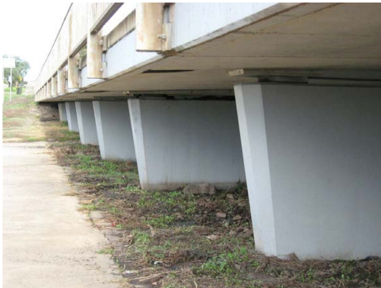
Figure 8 - Example Concrete Bridge Substructure (Pier Walls) Condition Score 1
