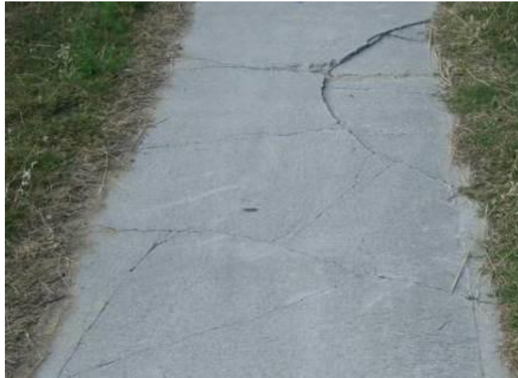
Figure 19 - Example Concrete Footpath Condition Score 5
