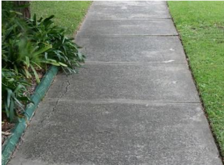
Figure 17 - Example Concrete Footpath Condition Score 3
