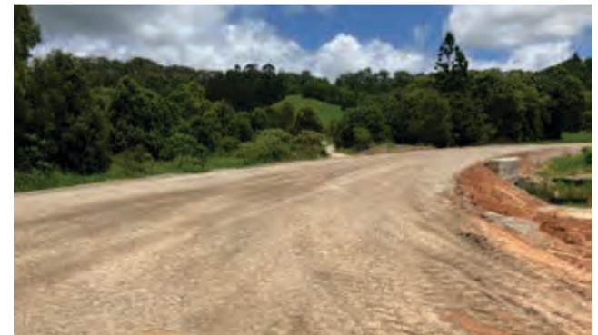
Crushed concrete has been used in the construction of an internal haul road at Stotts Creek Resource Recovery Centre.
