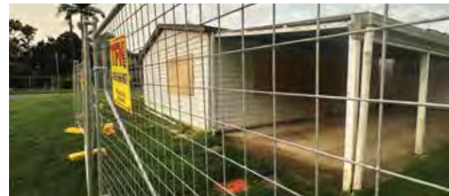
A flood-affected home is fenced off for a buyback.
