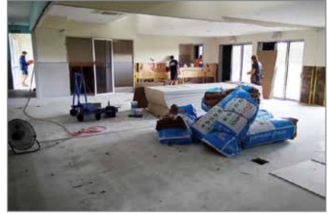
Contractors working on the internal walls of the Murwillumbah Community Centre.
