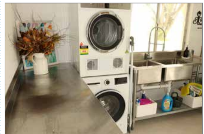
Stainless steel benches and having laundry equipment positioned to be raised case of future floods are part of the resilience measures taken at the Belle Riverhouse at Tumbulgum.
