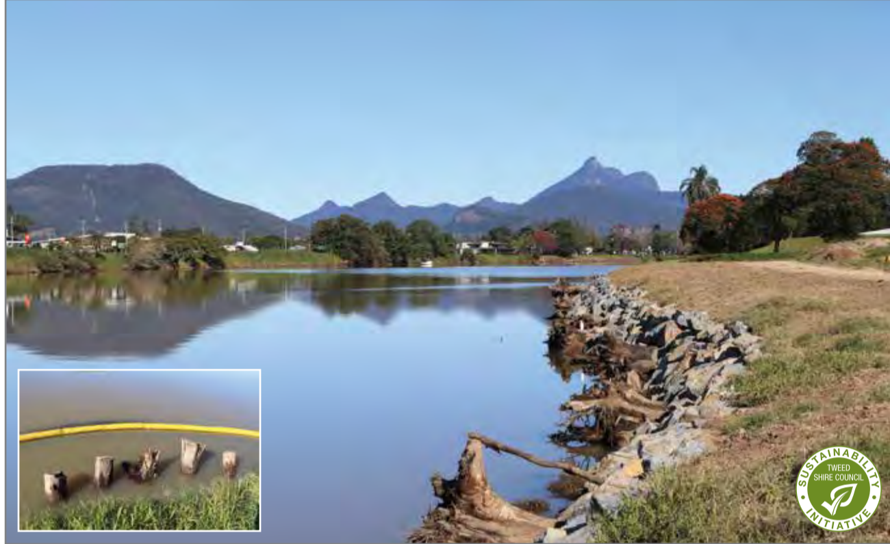
Eucalypt root balls and rock placed on the river bank at Murwillumbah to prevent further erosion and to provide fish habitat. Inset: Logs installed to stabilise the river bank along the Tweed River at Murwillumbah.
