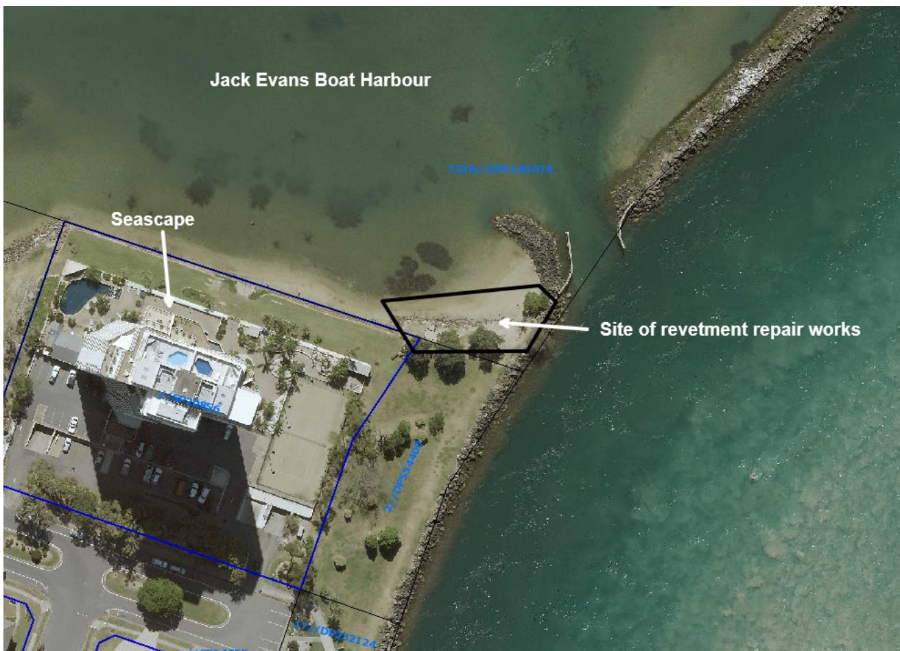
Figure 1: Site of revetment repair works
