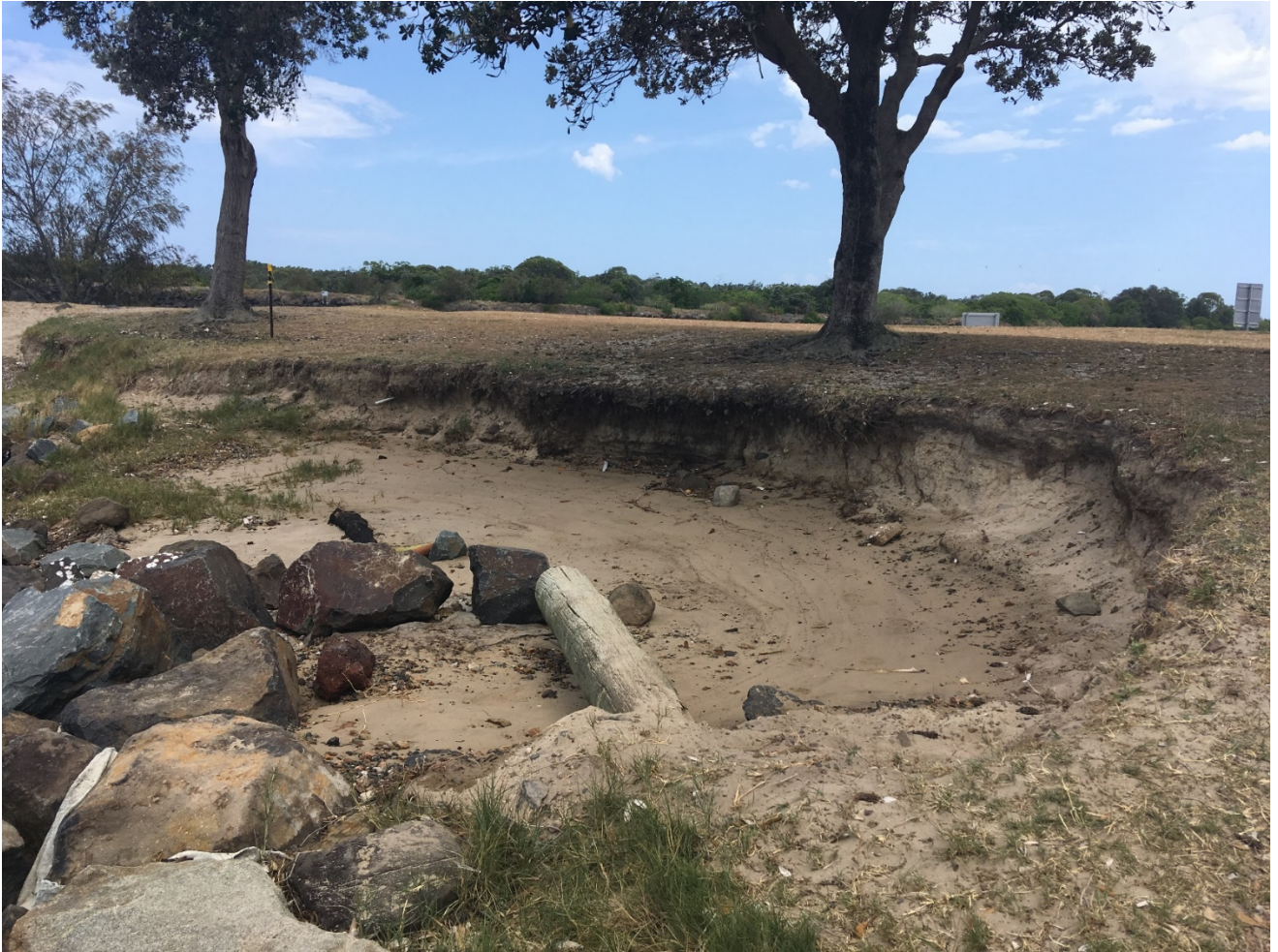
Figure 2: Erosion at the site illustrating the risk presented by the undermining of the trees
