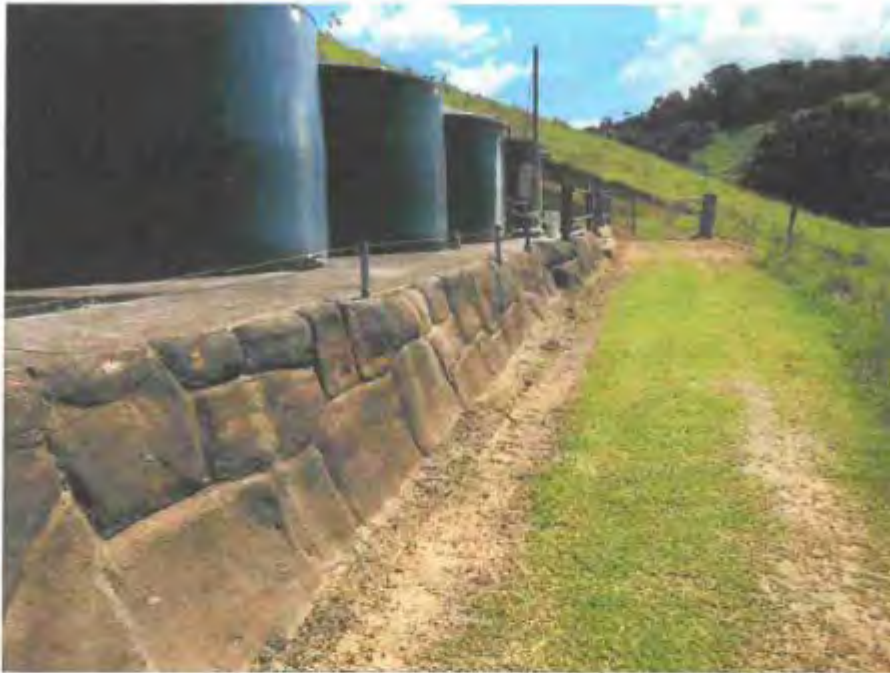
Figure 3 – Front retaining wall of tanks slab
