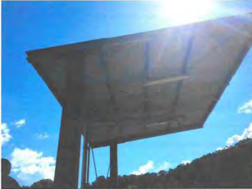
Figure 1 – Filling Station awning roof
