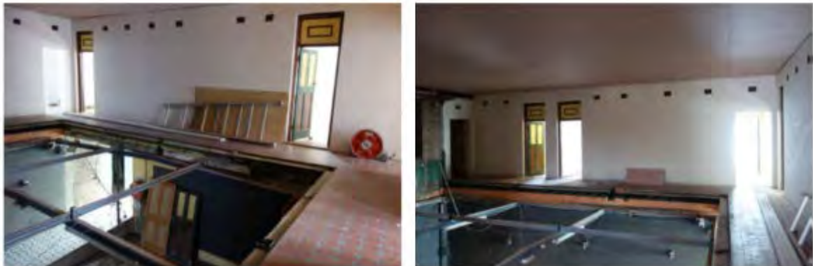
Figure 7: Existing Void area, with roof above as approved under DA17/0128
