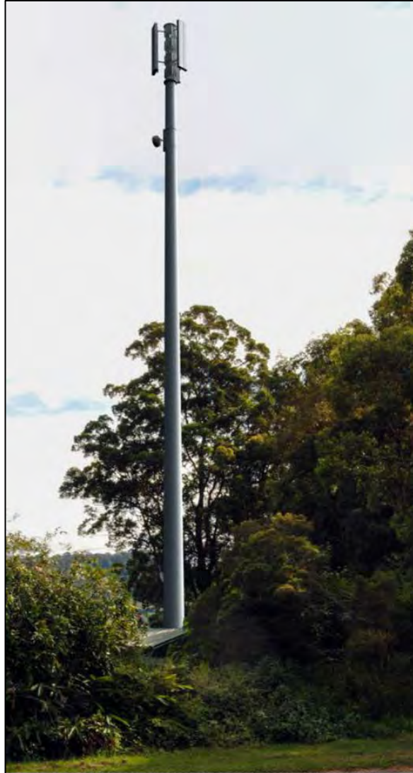
Figure 8: Photo montage of proposed facility (unpainted) when viewed from junction of Park Avenue/North Arm Road (View 6)
