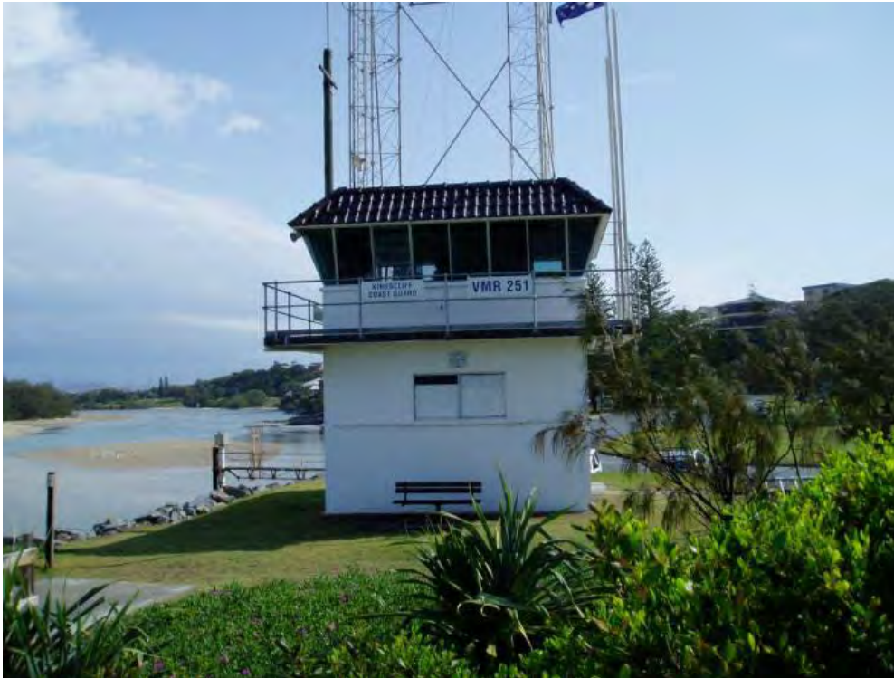
Photograph 1: AVCGA Kingscliff Flotilla Communications Tower
