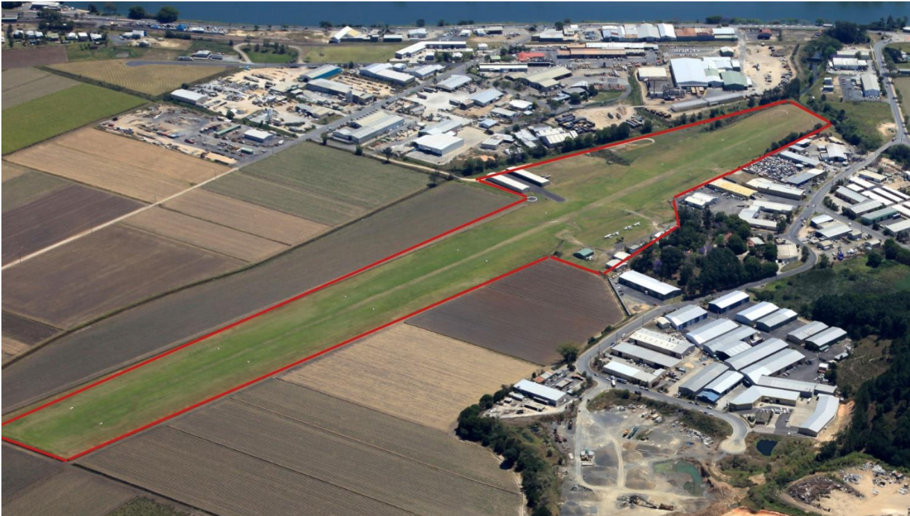
Figure 1 Aerial view of the Bob Whittle Murwillumbah Airfield
