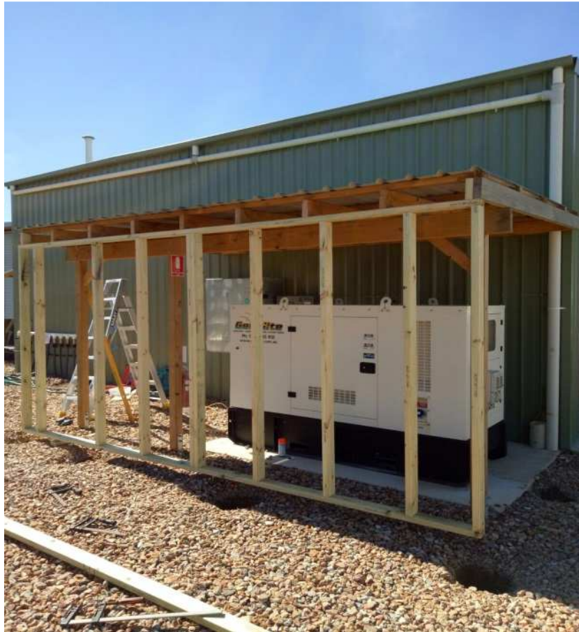
Generator being Noise Insulated
