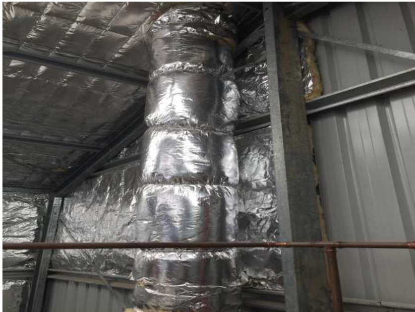
New Chimney Noise Insulated
