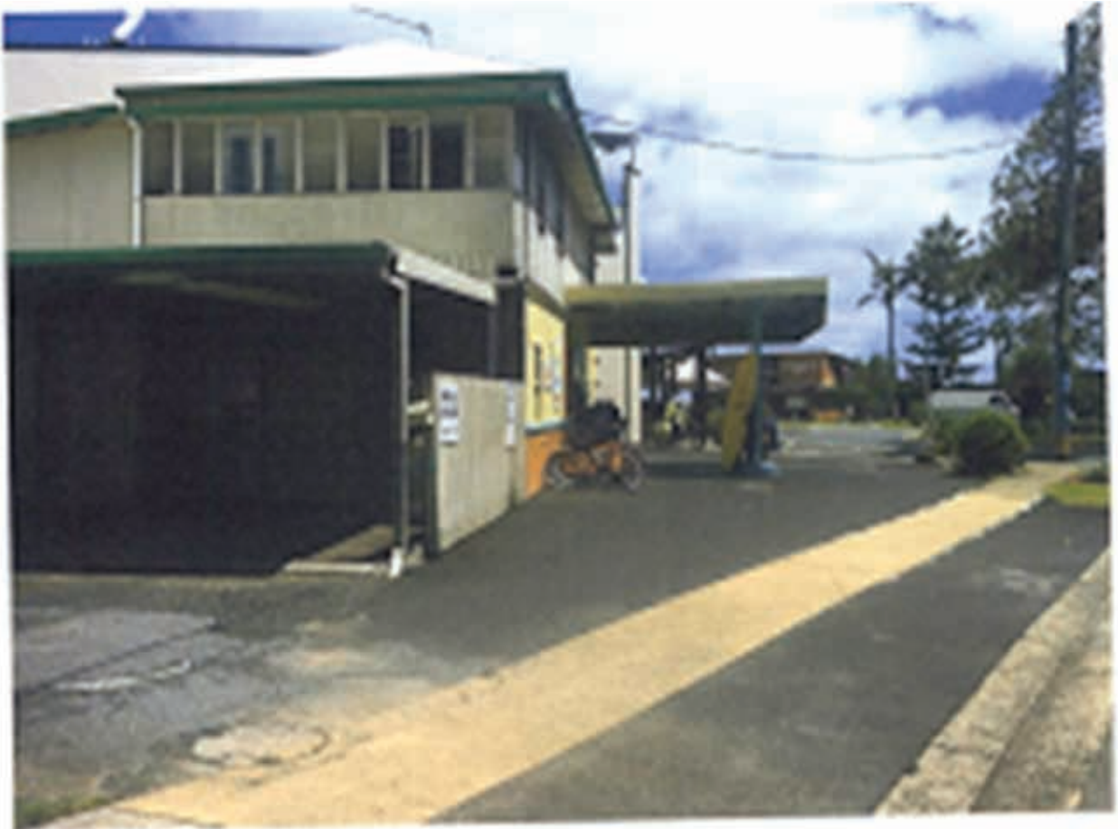
Photo from 17 January 2012 – after BP vacated the premises
