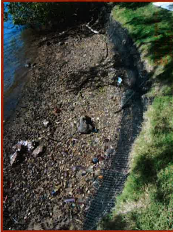
Figure B33 Soft armouring with geogrid and compost-filled mesh containers
