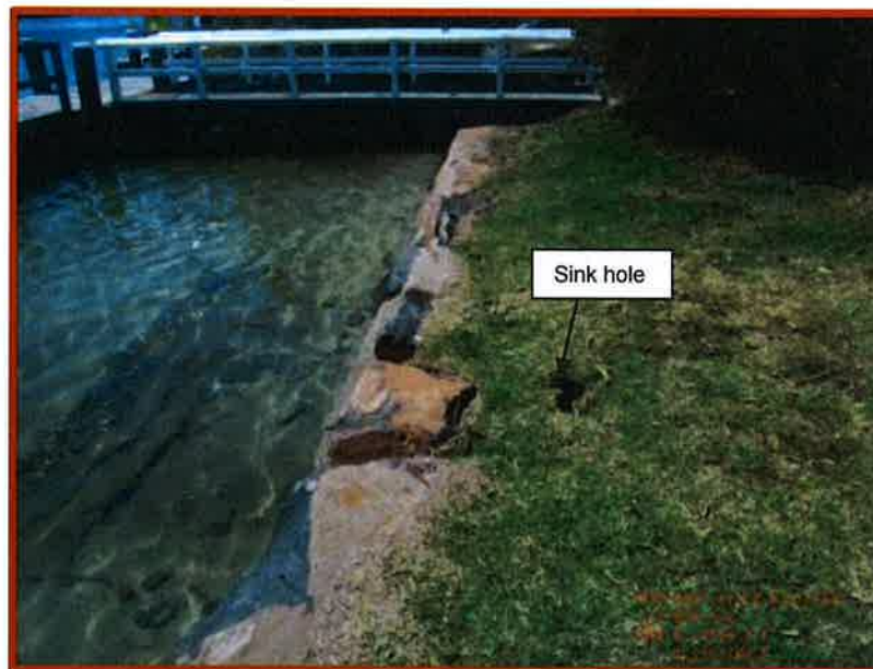
Figure B26 Vertical seawall adjacent to boat shed
