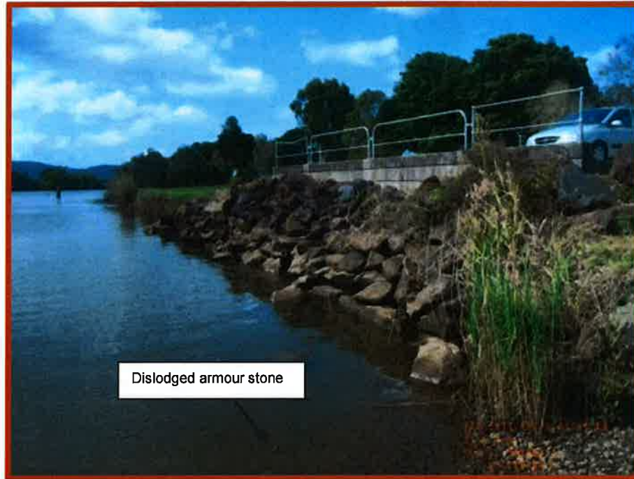
Figure B8 Revetment adjacent to boat ramp at Condong
