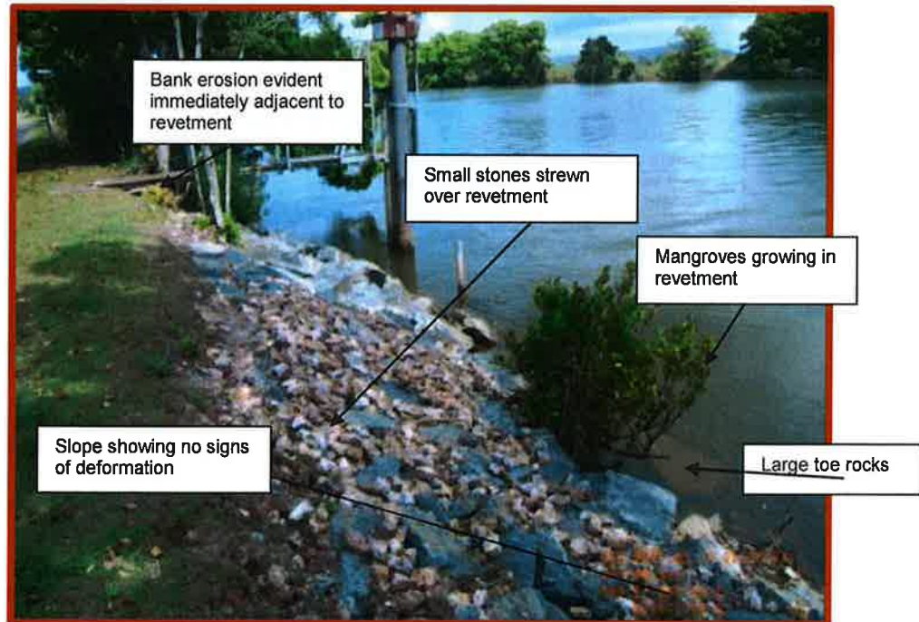
Figure B4 Revetment at Tumbulgum foreshore, looking west
