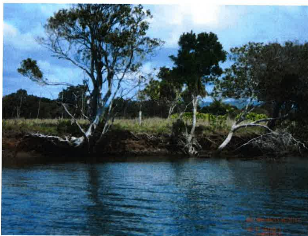
Figure A11 Photograph of an example section of river bank experiencing erosion resulting in a loss of riparian vegetation within the Tweed River.
