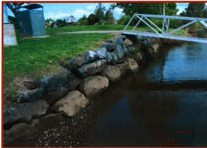
Figure B9 Seawall on upstream side of boat ramp at Condong
