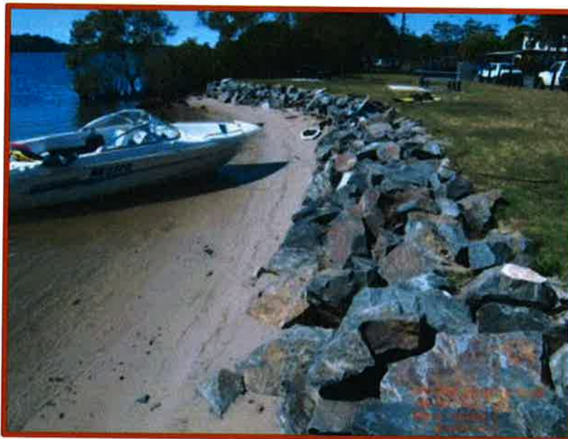
Figure B32 Typical new revetment section, Chinderah
