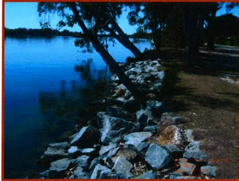
Figure B24 Philp Parade, with newly constructed revetment
