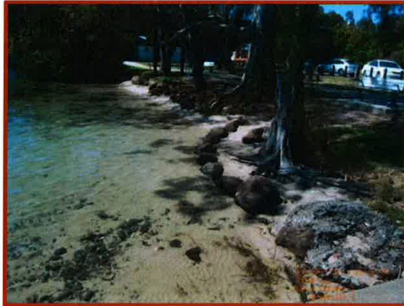
Figure B27 Rock protection for trees east of boat ramp at Dry Dock Road
