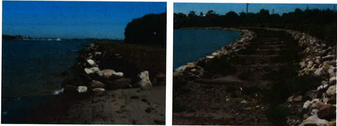
Figure 32 Moderate erosion along low bank (left) and possible solution* e.g. Claydon Reserve at Kogarah bay from DECCW, 2009 (right)
