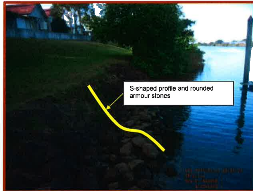
Figure B18 Revetment at Heritage Wharf
