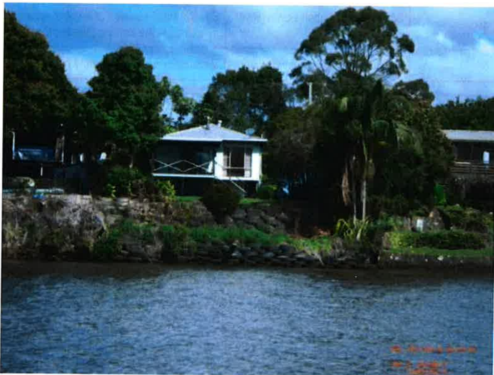
Figure A15 Photograph of an example section of river bank demonstrating the variable river bank defence structures implemented along private land, with a concrete seawall joining up to a tyre seawall.
