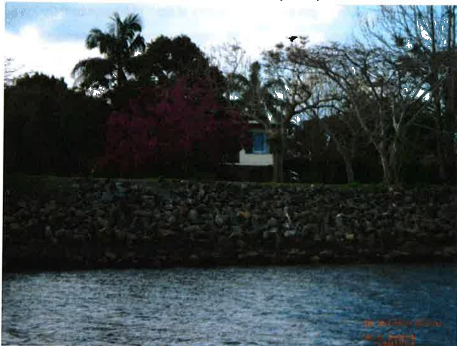
Figure 33 Well designed rock revetment (Tweed River)
