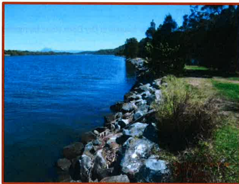
Figure B29 Revetment at Oxley Cove (west)
