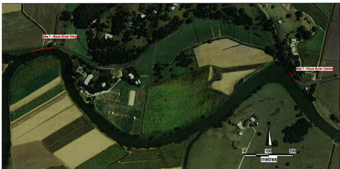
Figure B19 Road embankment protection at Rous River
