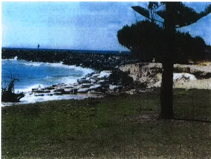
Figure 9 - Looking south from Faulks Park following erosion events of 2010. Also evident are the end effects of Cudgen Creek training walls. Photo: B Gibbs 12 August 2010.
