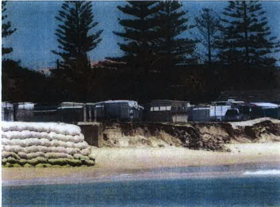
Figure 12 – Looking towards the Holiday Park showing end effects of temporary protection works and the current risk posed to the amenities block and pumping station located immediately behind the escarpment. Photo: G Pezzimenti 8 November 2011.
