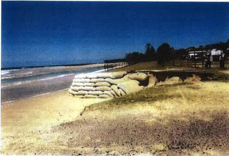
Figure 10 - Northern end of the geotextile sandbag seawall (looking south) showing both collapse of the wall and end effects which have produced further erosion of the Holiday Park. Photo: M Daley 8 November 2011.
