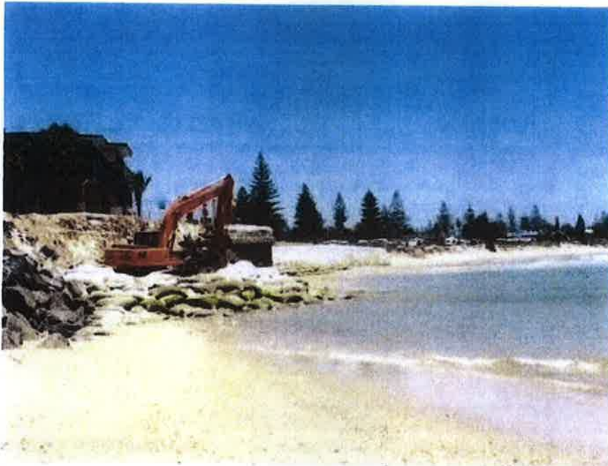
Figure 7 - Looking north from the terminal rock revetment towards Cudgen Headland SLSC and the Holiday Park showing both the piled concrete foundations and temporary geotextile sandbag wall. Photo: M Daley 8 November 2011.
