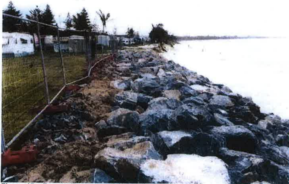
Figure 15 – Recent (December 2011) rock revetment works installed to protect the amenities block and sewer pumping station of the Kingscliff Holiday Park. Photo: B. Fitzgibbon 14 December 2011.
