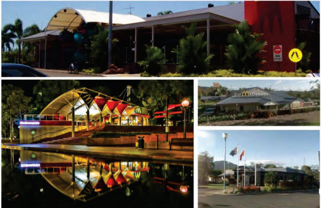
McDonald's restaurants displaying some climatically appropriate design measures including deep verandas, eaves, varying roof forms and internal volumes and references to regional architecture.
