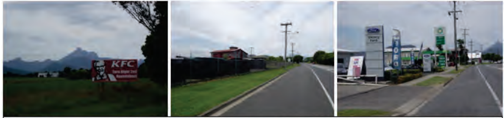
Poor Entrance sequence elements into Murwillumbah includes signage tainting view fields, long stretches of wire-mesh-fencing and a limited amount of significant landscape or mature trees. ¶
