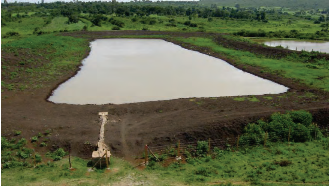
Figure 1. The rehabilitated Gona Dam, recently filled
