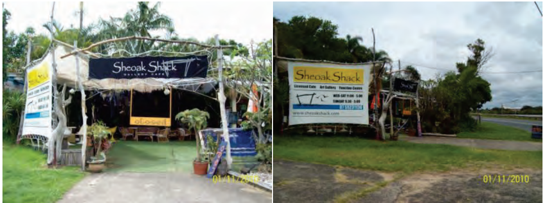
Figure 2: Existing structures at entrance of Sheoak Shack
