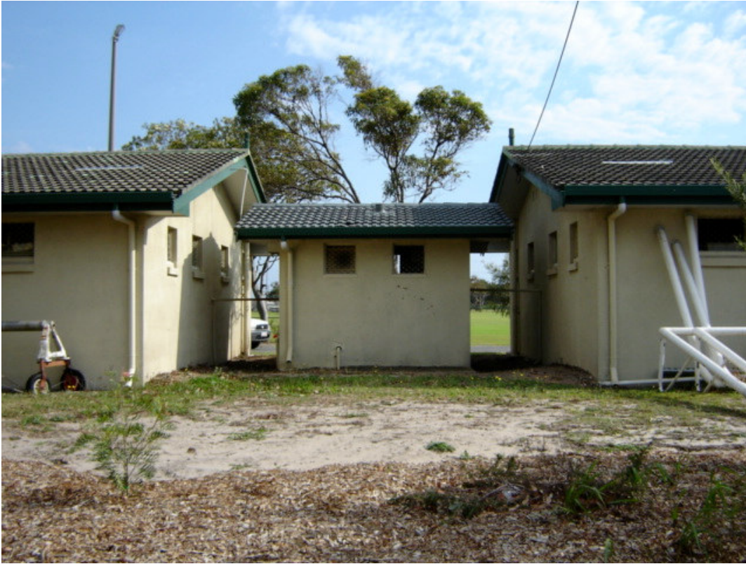
Figure F7 Reg Dalton Oval Existing Amenities Buildings & Existing Bore Pump Shed (centre)
