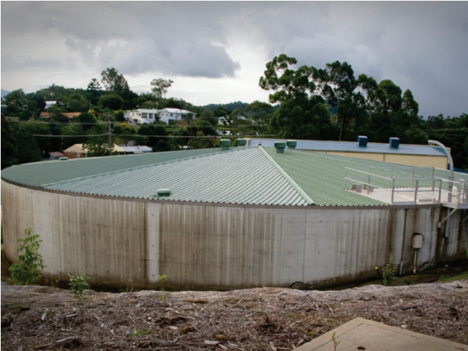
Clear Water Tank
