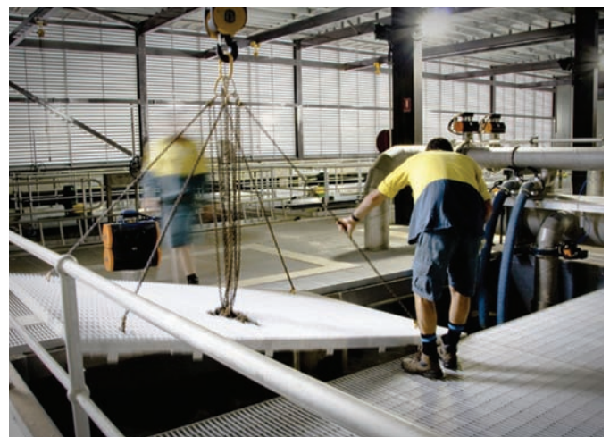
Staff removing grate to remove membranes
