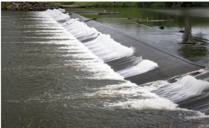
Bray Park Weir
