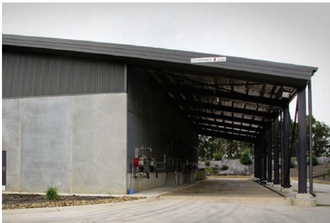
Chemical Storage Facility
