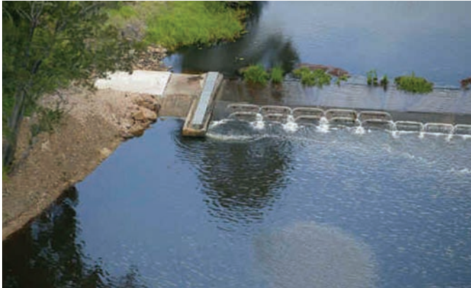
Bray Park Weir
