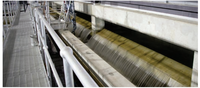
Pre-flocculation Tank
