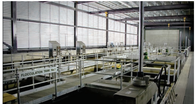
Flocculation Tanks
