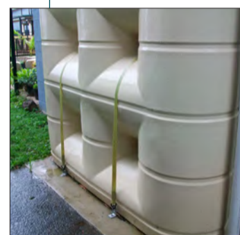
Water tank strapped down to slab, which is poured and reinforced into main slab.
