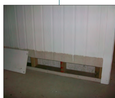
Removable skirting board allows framework to be flushed clean of silt. Timber framework below flood level is H3 treated timbers for water resistance and noggins above have holes drilled in them to allow the frame to easily drain. The wall lining is cement sheet for water resistance. White walls were easily cleaned the day after flood waters receded using a product like 30 Seconds and then pressure cleaned.
