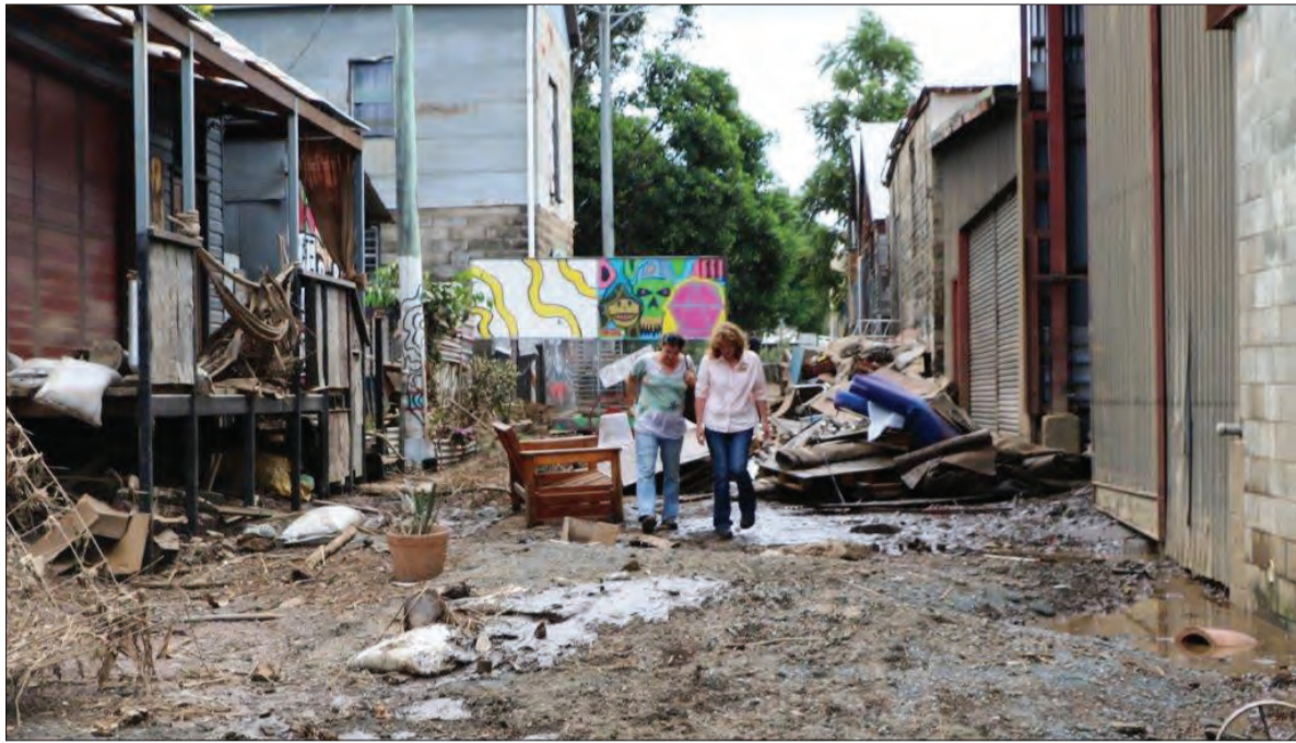
Above: Holstons Lane in South Murwillumbah shows the damage a flood can wreak on both residential houses and businesses.
