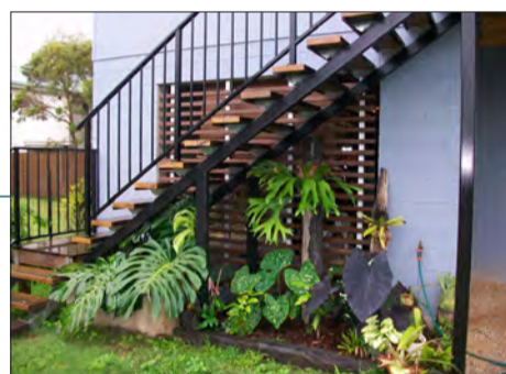
Secure flood openings with 65 per cent openness – H3 treated timber fixed to galvanised supports. Easy wash out under.
