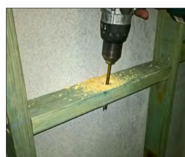
Removable skirting board allows framework to be flushed clean of silt. Timber framework below flood level is H3 treated timbers for water resistance and noggins above have holes drilled in them to allow the frame to easily drain. The wall lining is cement sheet for water resistance. White walls were easily cleaned the day after flood waters receded using a product like 30 Seconds and then pressure cleaned.
