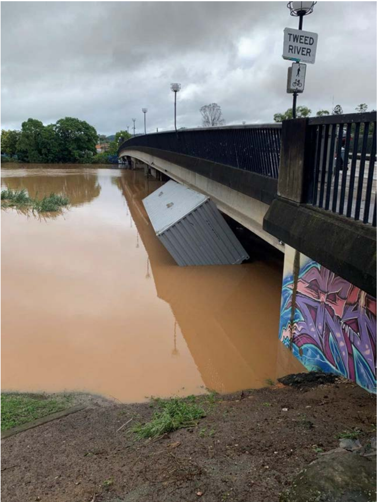
Upstream side of Murwillumbah bridge looking west
