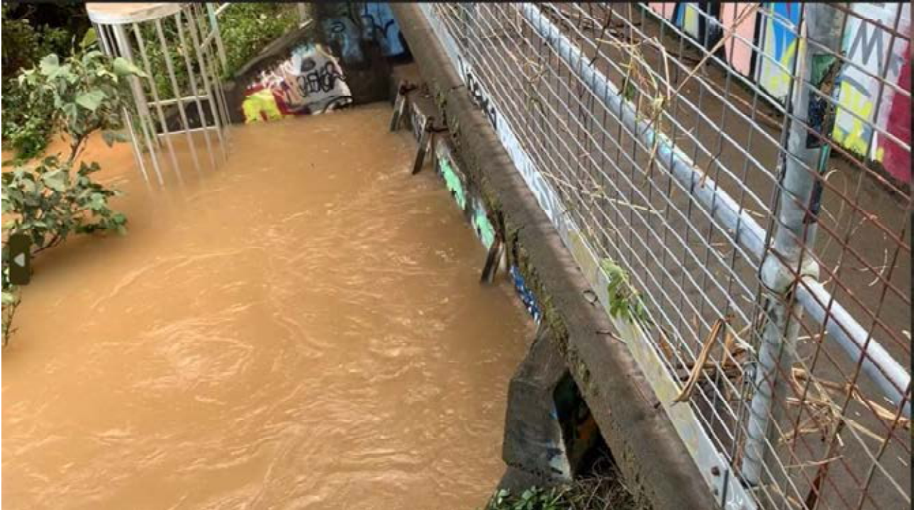
Outlet of Lavender Creek pumps
