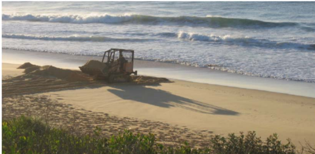
Figure 3-1 Beach Re-profiling using Mechanical Equipment (Souce: Carley et al., 2010)
