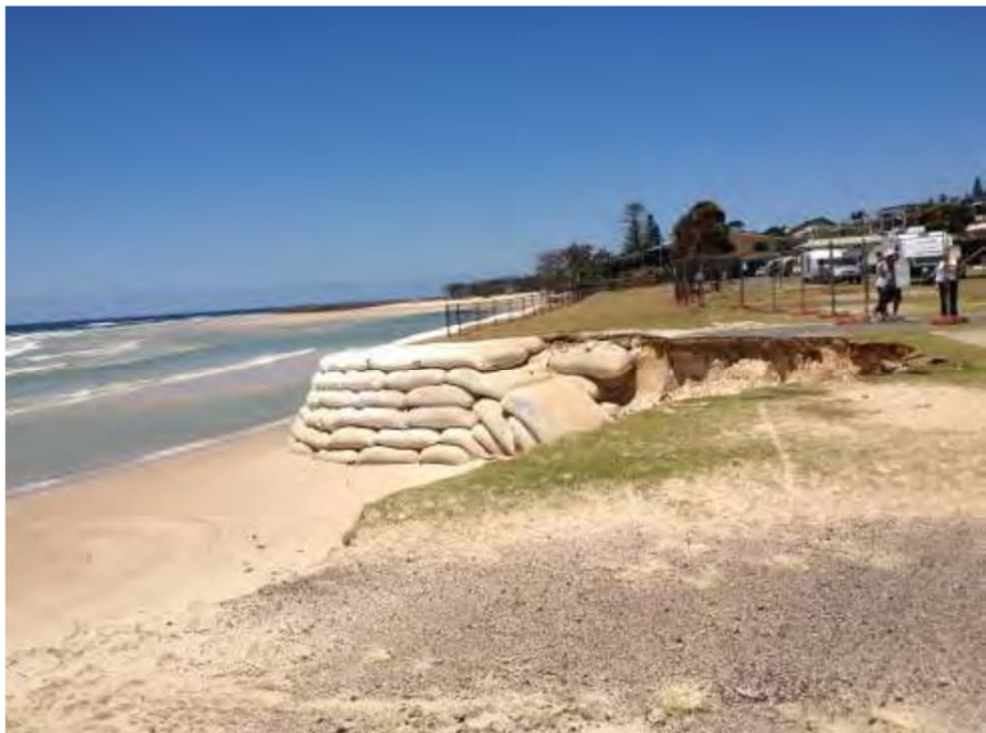
Figure 3-3 End Effects at Geotextile Sand Container Wall at Kingscliff Beach Holiday Park (from NSW Government, 2011)
