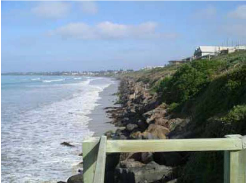
Figure 3-2 Seawalls on Eroding Shorelines Cause Loss of Usable Beach
