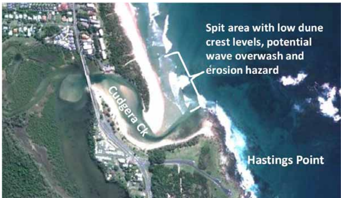
Figure 5-11 Zone of wave overwash and coastal entrance instability – Cudgera Creek
