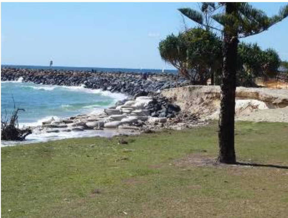
Figure 9 - Looking south from Faulks Park following erosion events of 2010. Also evident are the end effects of Cudgen Creek training walls. Photo: B Gibbs 12 August 2010.
