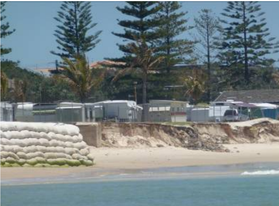
Figure 12 – Looking towards the Holiday Park showing end effects of temporary protection works and the current risk posed to the amenities block and pumping station located immediately behind the escarpment. Photo: G Pezzimenti 8 November 2011.
