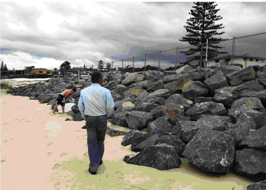
Figure 11 – Most recent (60 metre) rock extension in front of the further part of the Holiday Park and the amenities block. Photo: B. Fitzgibbon 14 December 2011.
