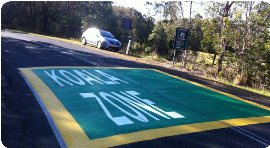
Figure 15: Tweed koala road variable message sign and pavement treatment
