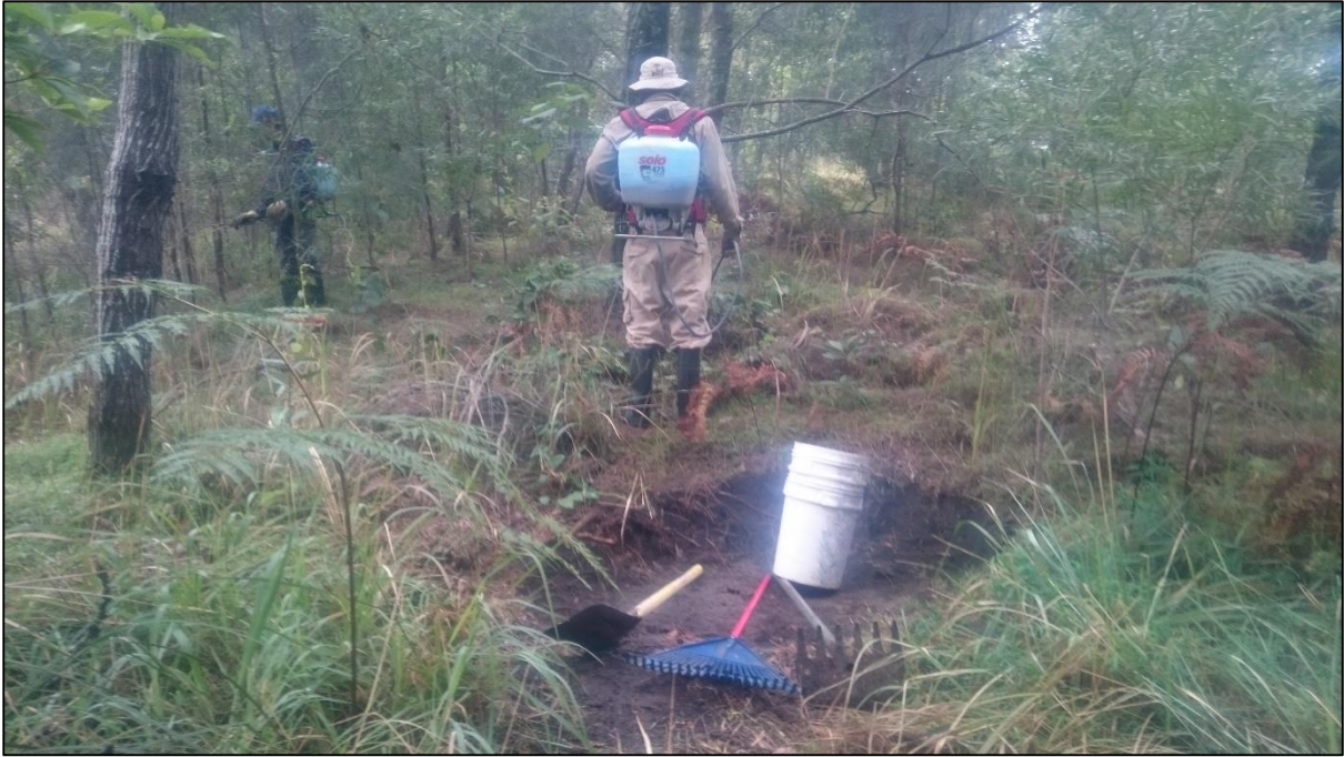
Tools and soil disturbed to construct bicycle track at "Glossy Black"
