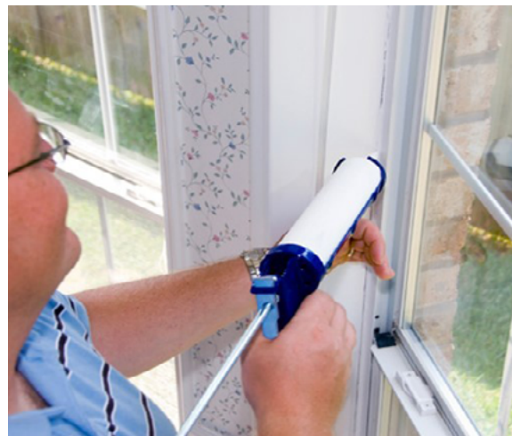
Sealing drafts can make homes more energy efficiency to heat and cool
