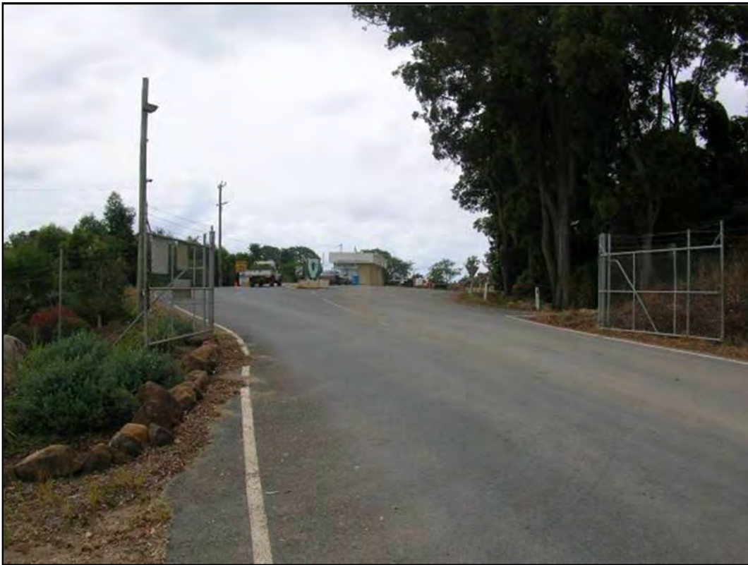
Figure 55 Site Access from Leddays Creek Road
