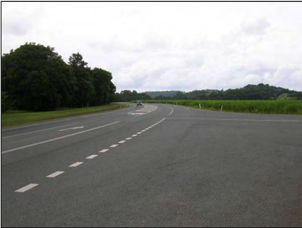
Figure 54 Tweed Valley Way from Leddays Creek Road Intersection
