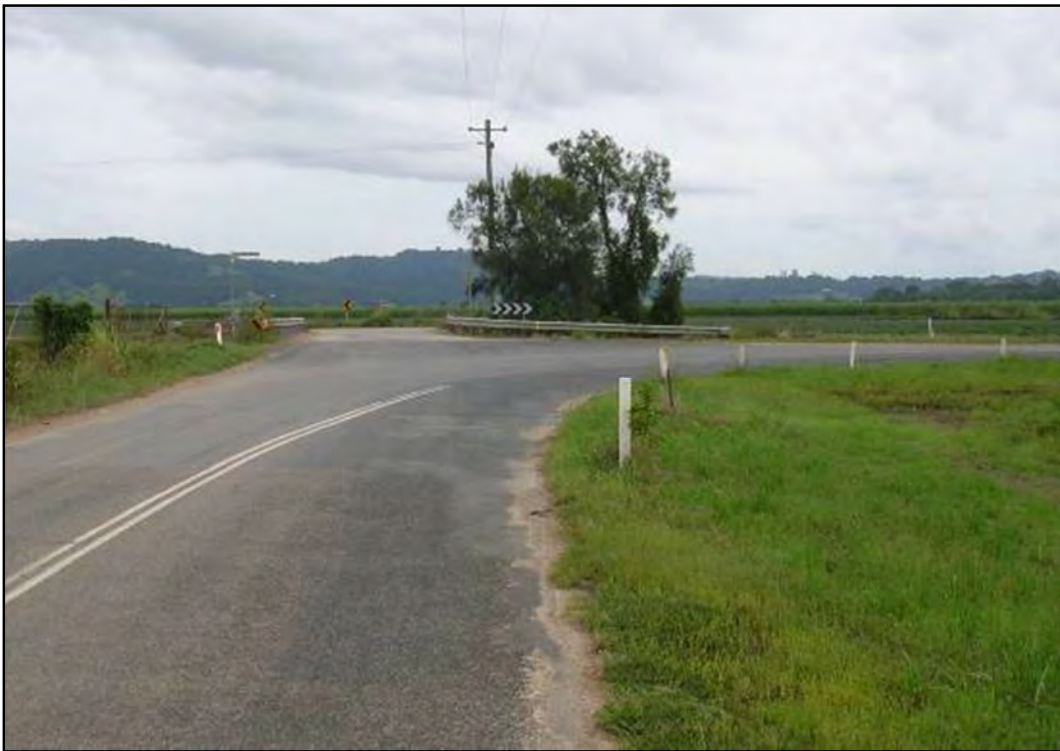
Figure 58 Intersection Leddays Creek Road (Site Access Road) and Bartletts Road
