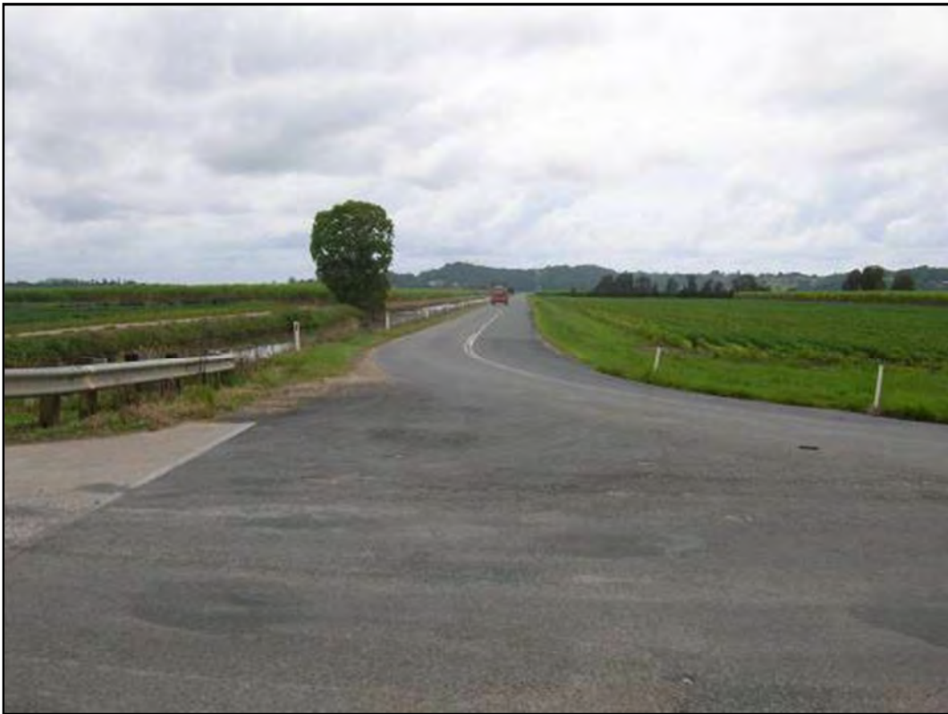
Figure 53 Leddays Creek Road Looking North from Bartletts Road Intersection
