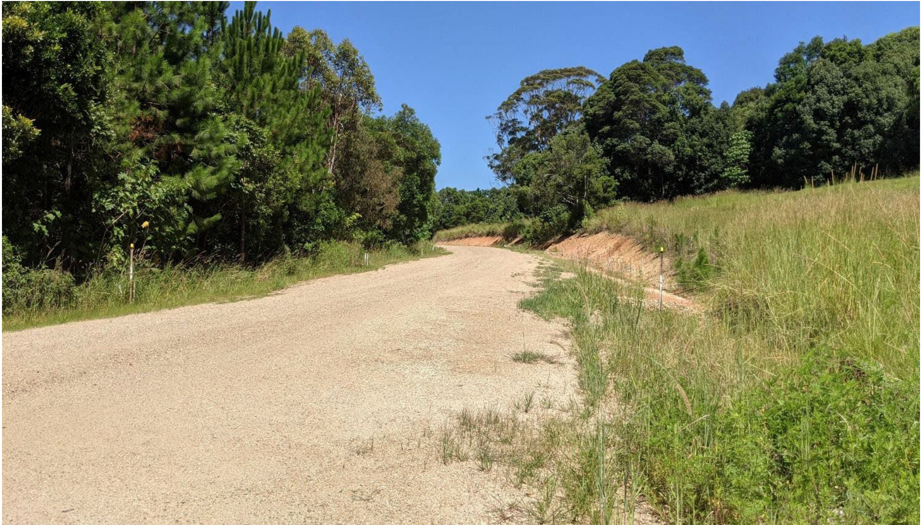
Figure 13: Material placed within haul road alignment looking south at approximately CH600
