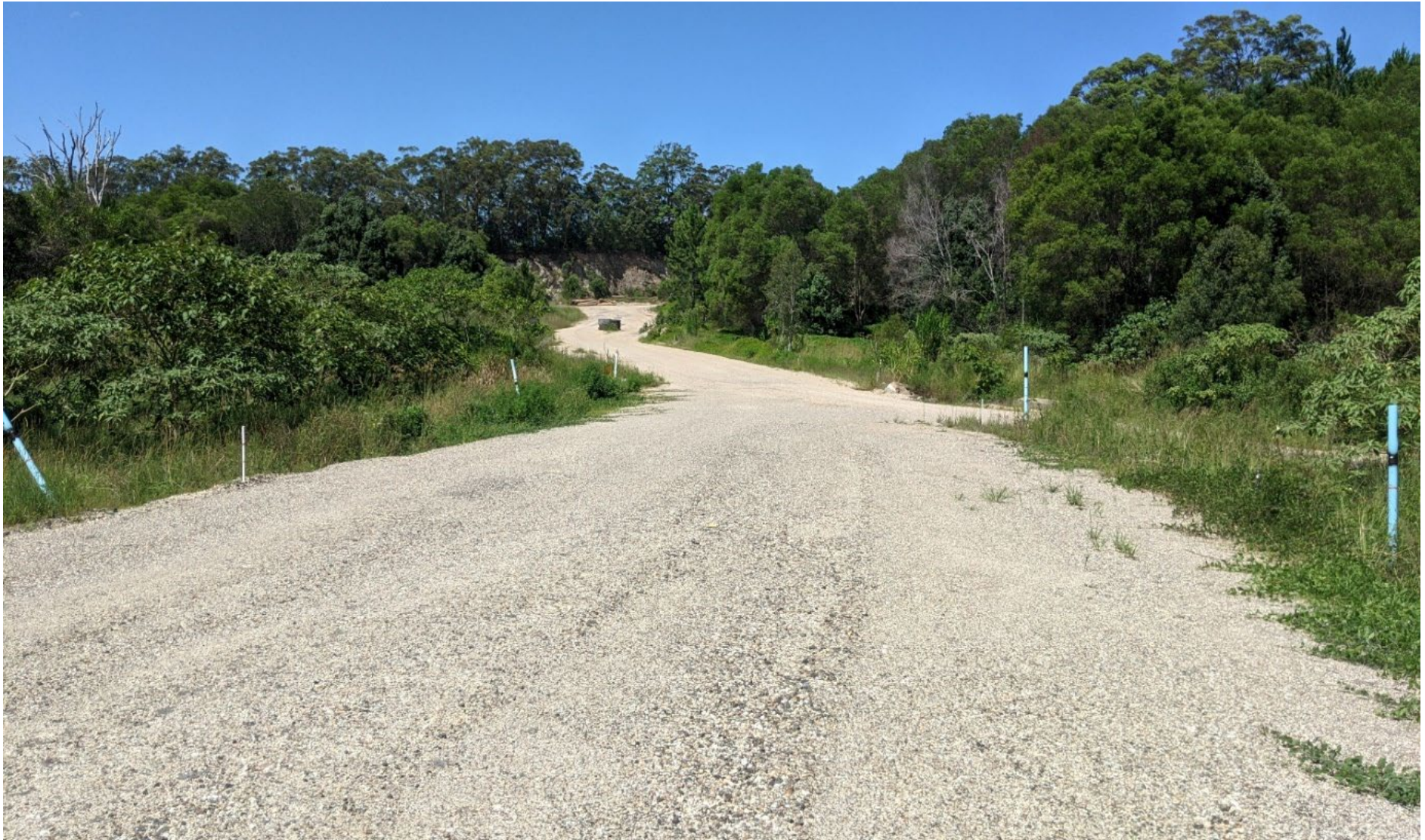
Figure 12: Material placed within haul road alignment looking east at approximately CH150
