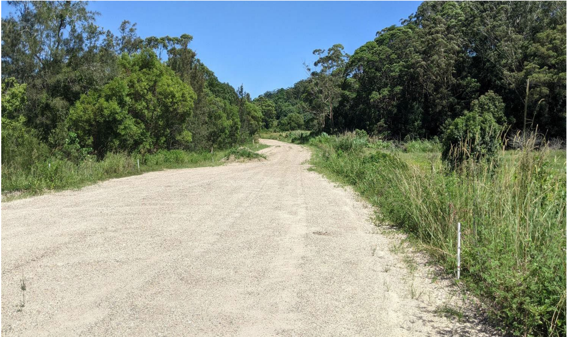
Figure 14: Material placed within haul road alignment looking south at approximately CH900
