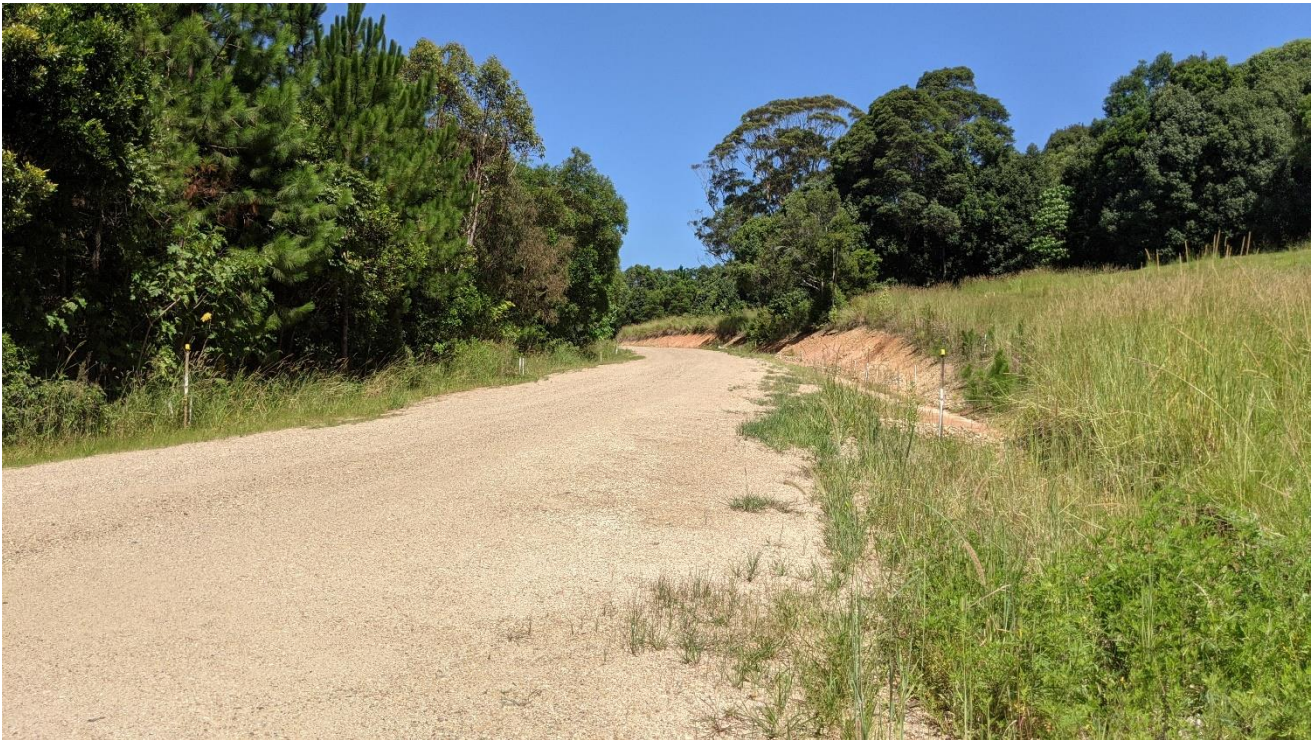
Figure 5: Material placed within haul road alignment looking south at approximately CH600.
