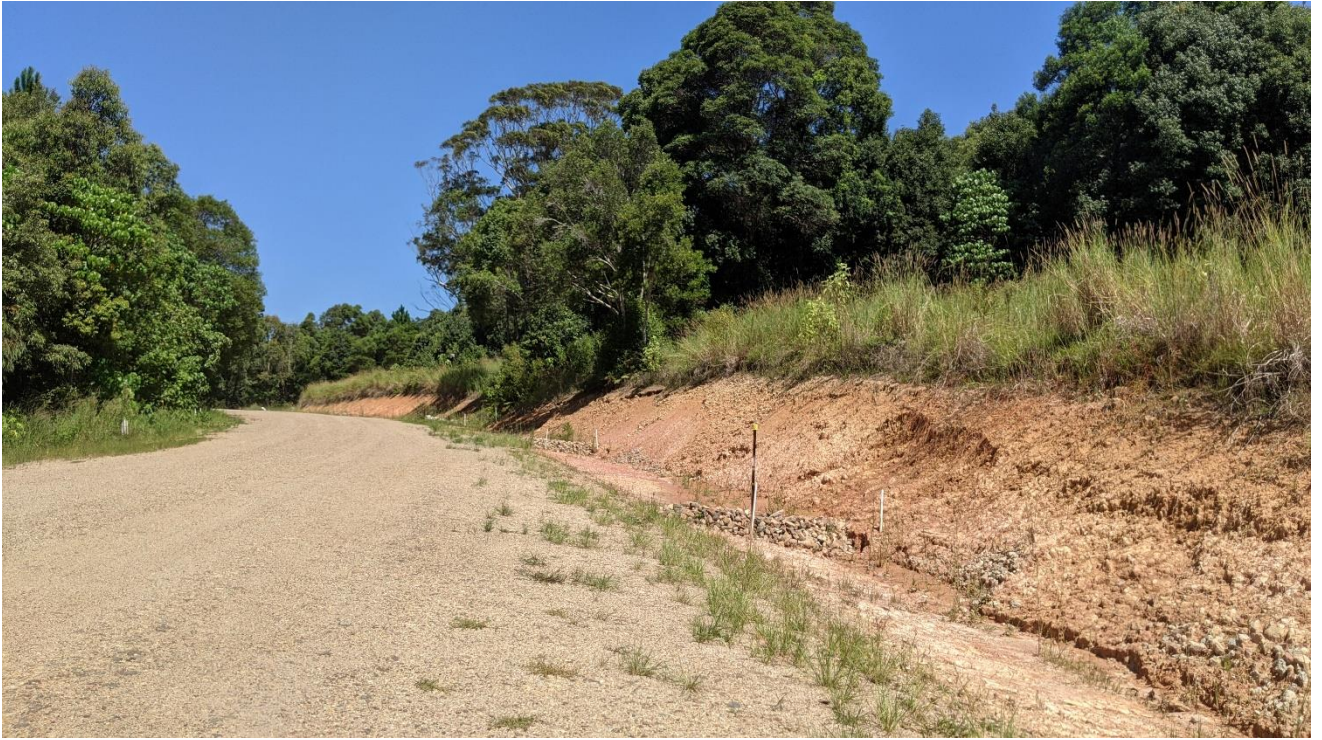
Figure 3: Rock check dams installed within table drains for erosion and sediment control.
