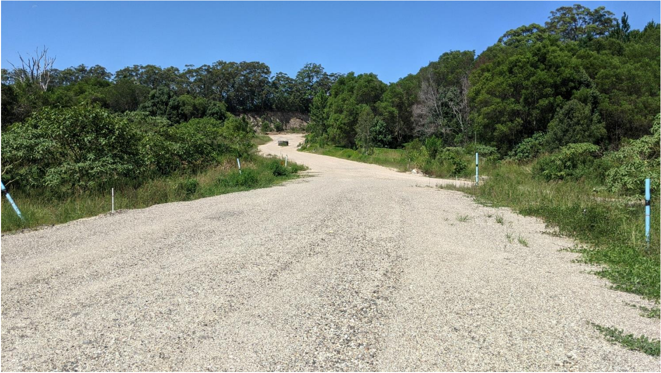
Figure 4: Material placed within haul road alignment looking east at approximately CH150.
