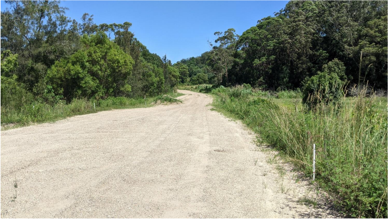
Figure 6: Material placed within haul road alignment looking south at approximately CH900.
