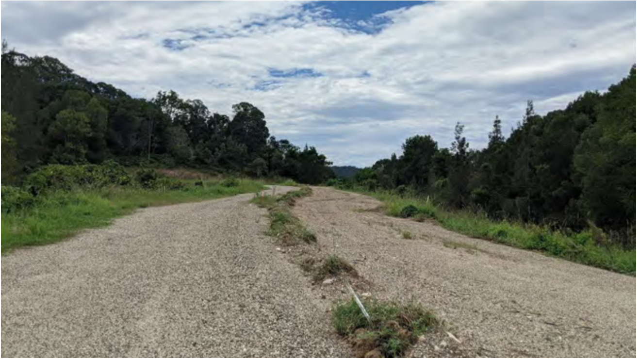
Figure 6: Material placed within haul road alignment looking north at approximately CH800.
