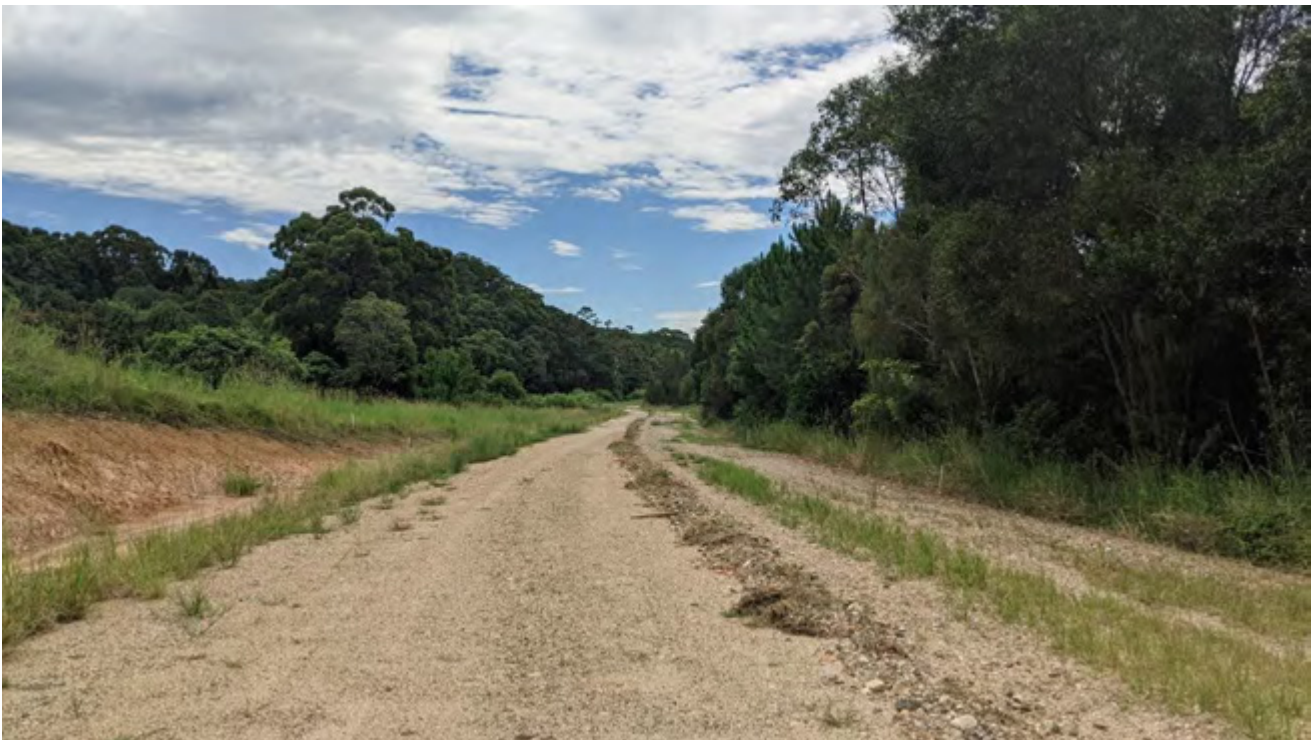
Figure 5: Material placed within haul road alignment looking north at approximately CH400.
