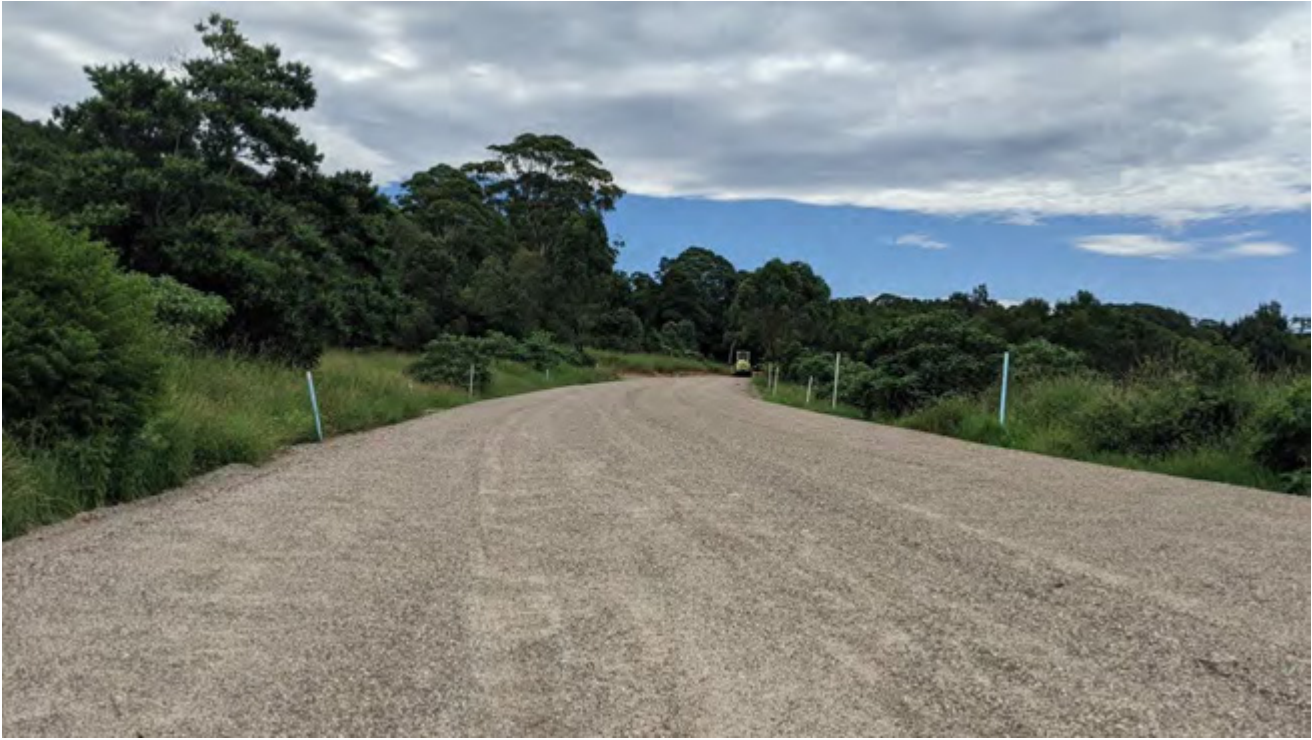
Figure 4: Material placed within haul road alignment looking north at approximately CH150.
