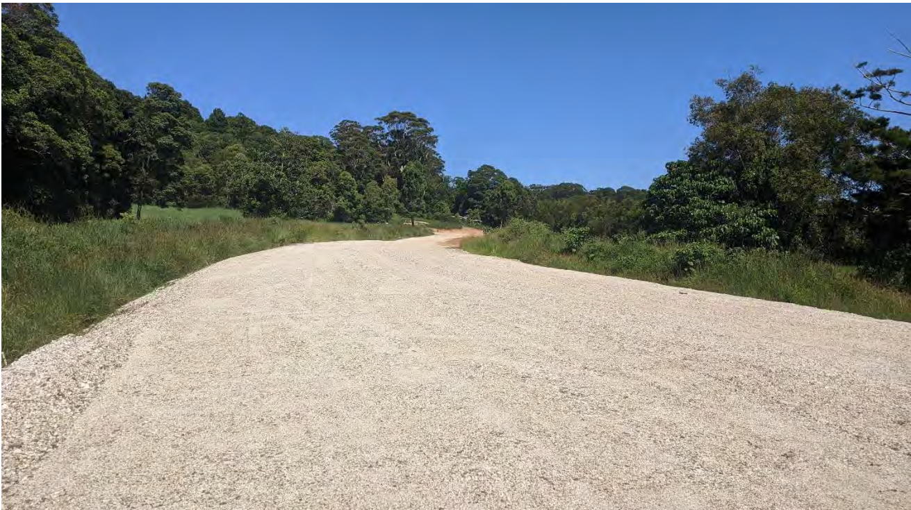
Figure 5 – Material placed within haul road alignment looking north at approximately CH150.
