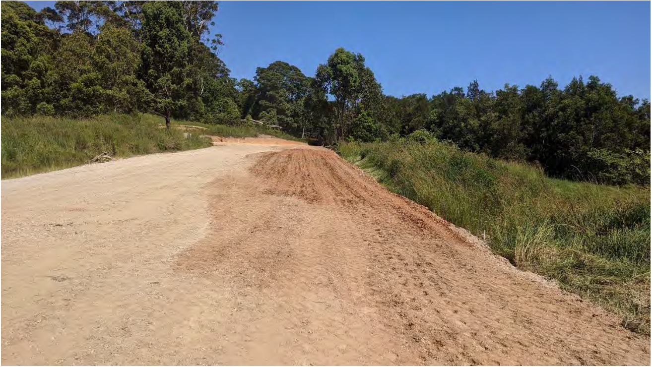
Figure 6 – Material placed within haul road alignment looking north at approximately CH280.
