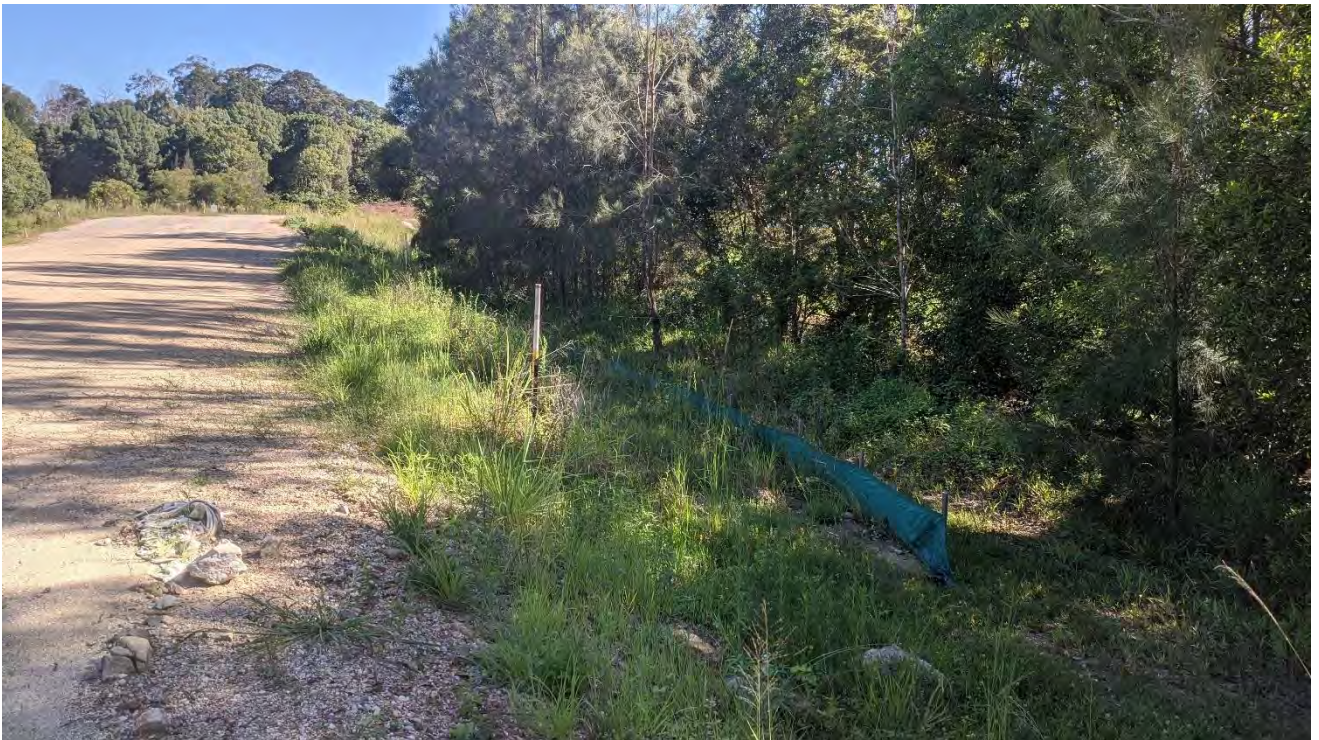
Figure 2 – Erosion and sediment controls adjacent exposed areas.
