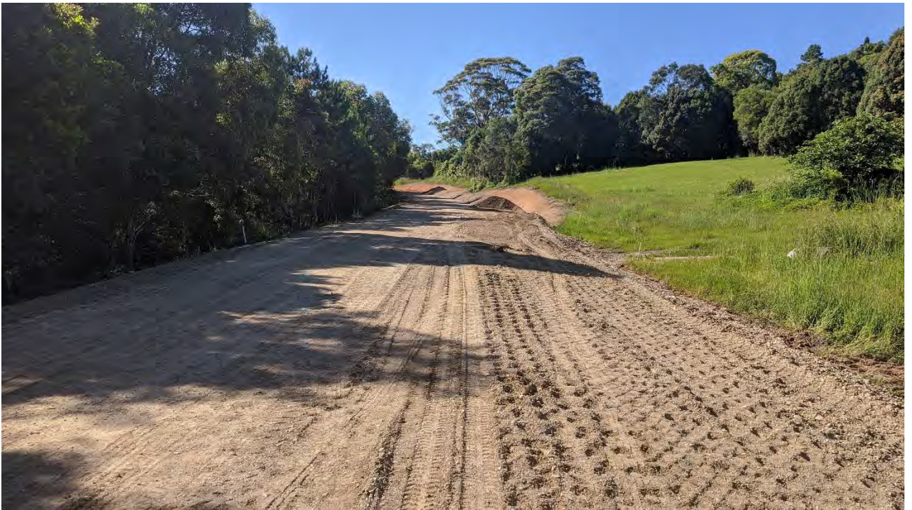
Figure 7 – Material placed within haul road alignment looking south at approximately CH600.
