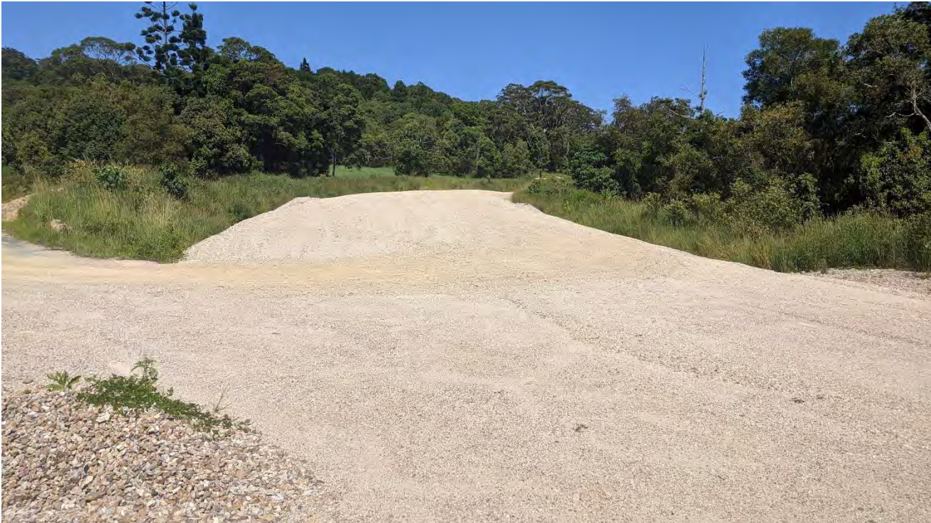
Figure 4 – Material placed within haul road alignment looking north at approximately CH50.
