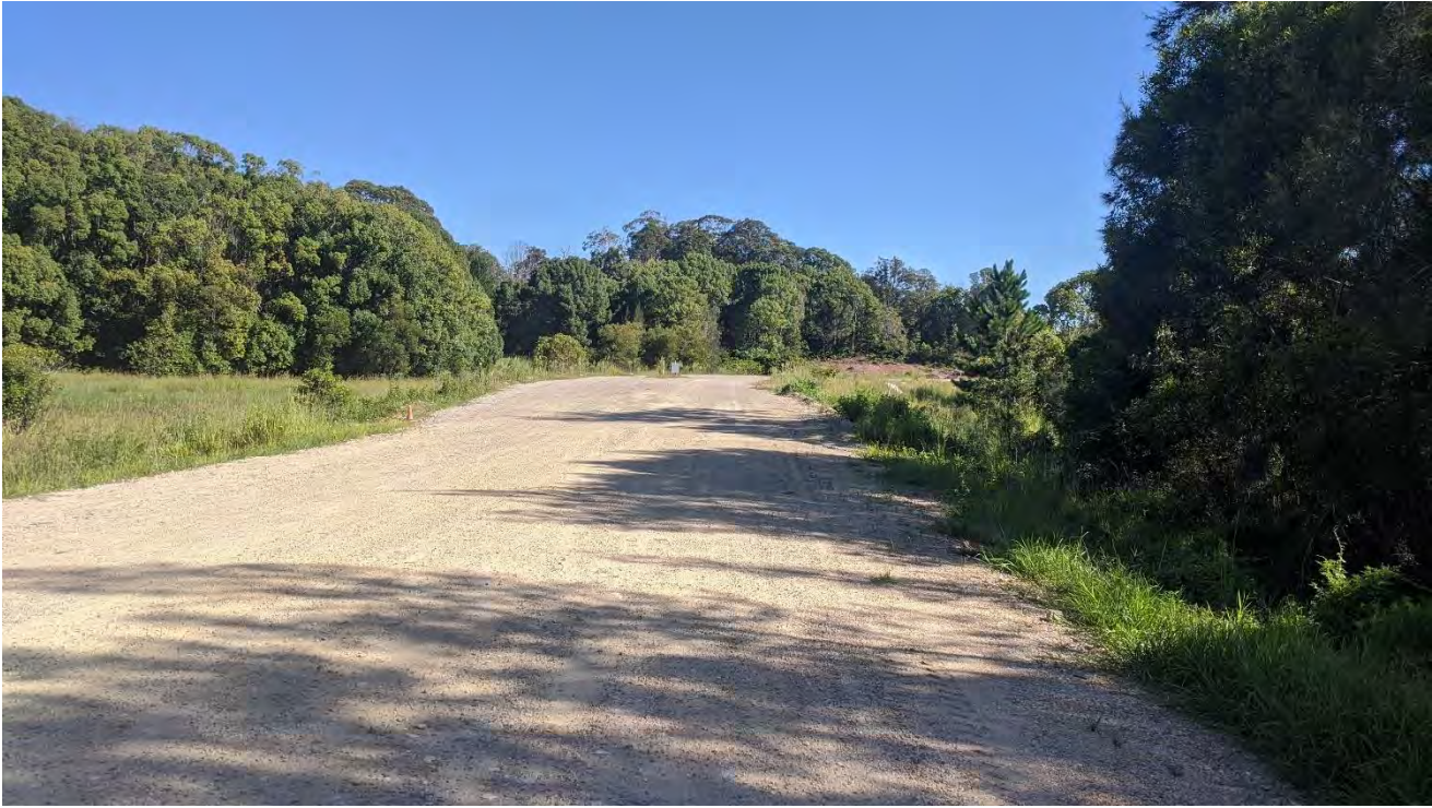
Figure 8 – Material placed within haul road alignment looking north at approximately CH800.
