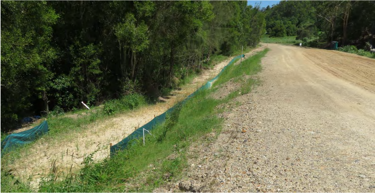
Figure 2 – Erosion and sediment controls adjacent exposed areas.
