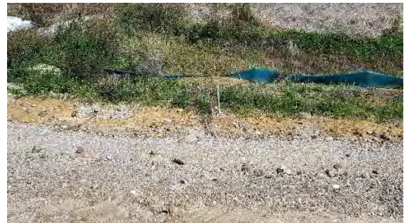
Photograph 6: Haul Road ErSED controls No. 3
