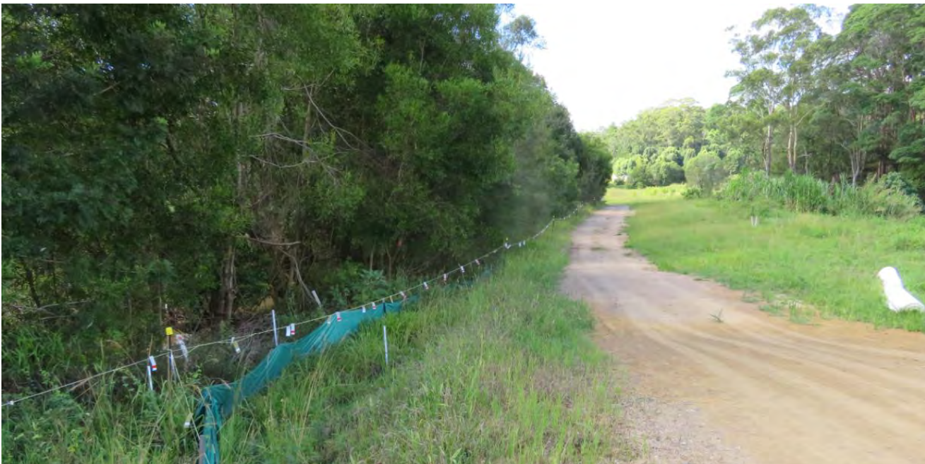
Figure 1 – Vegetation protection area and erosion and sediment controls.
