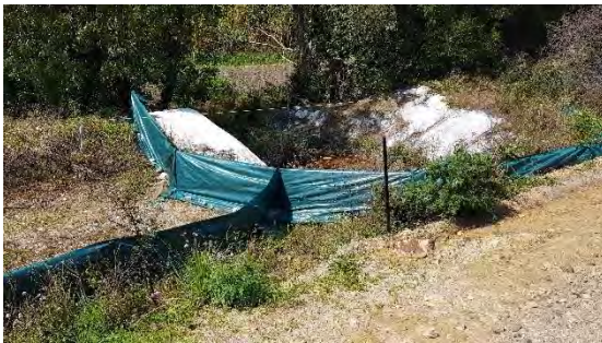
Photograph 5: Haul Road ERSED controls No. 2
