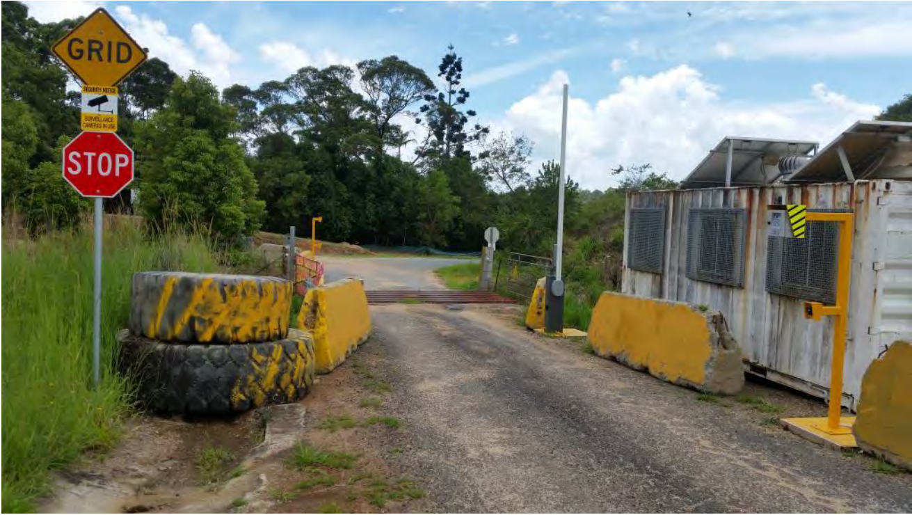
Figure 3 – Fob activated boom gate constructed at entrance to haul road site.
