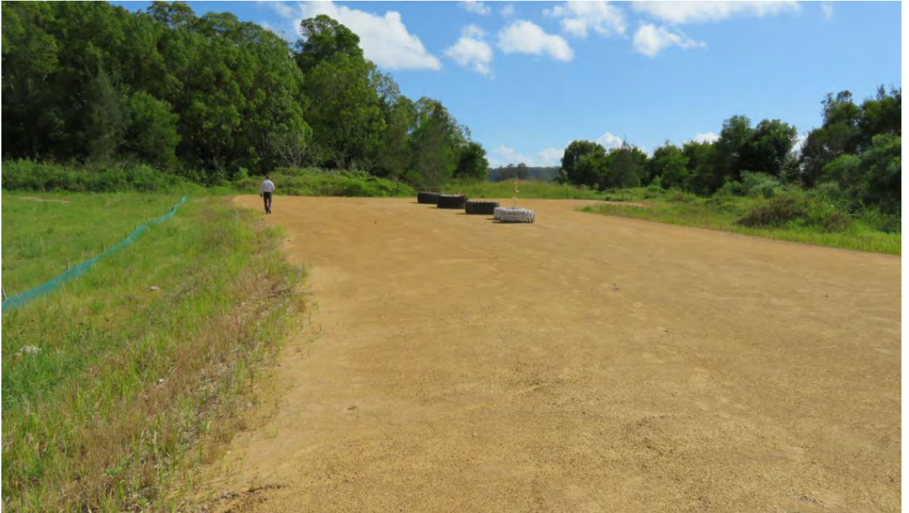
Figure 5 – Material placed within haul road alignment between approximately CH800 and CH1000.
