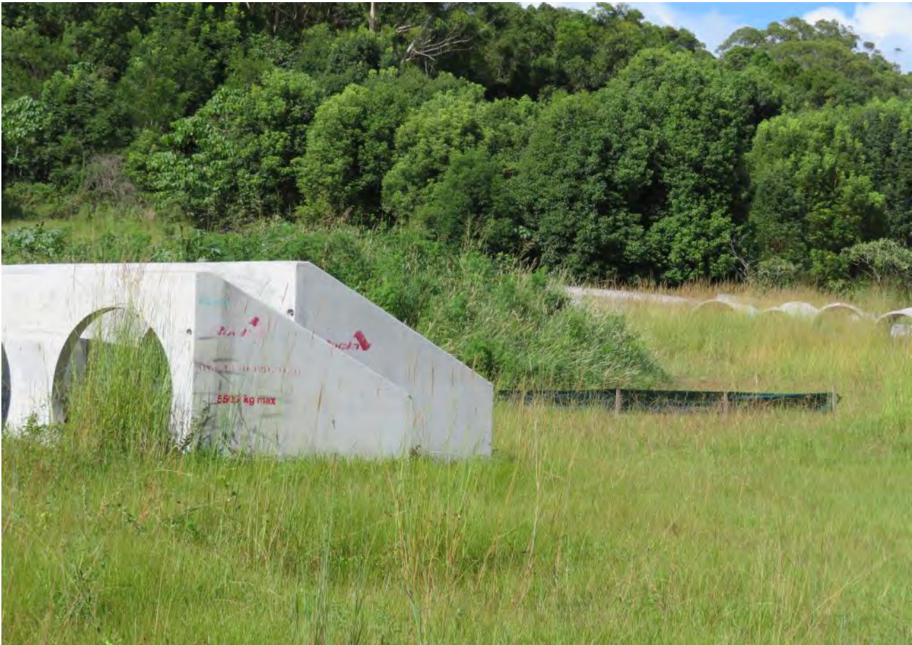
Figure 4 – Photo of vegetated stockpiles and stormwater infrastructure on site ready for installation.
