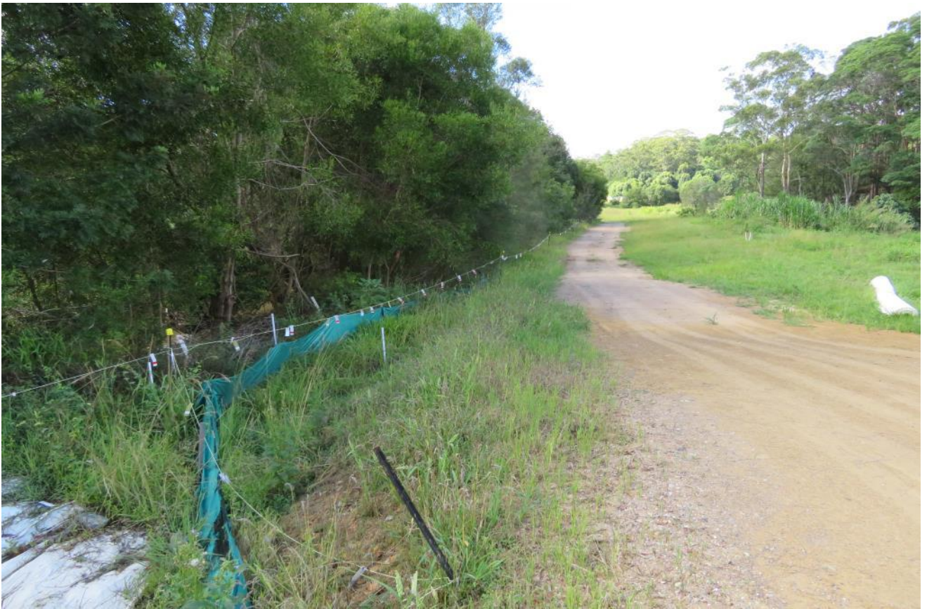
Figure 5 – Environmental controls along haul road alignment.
