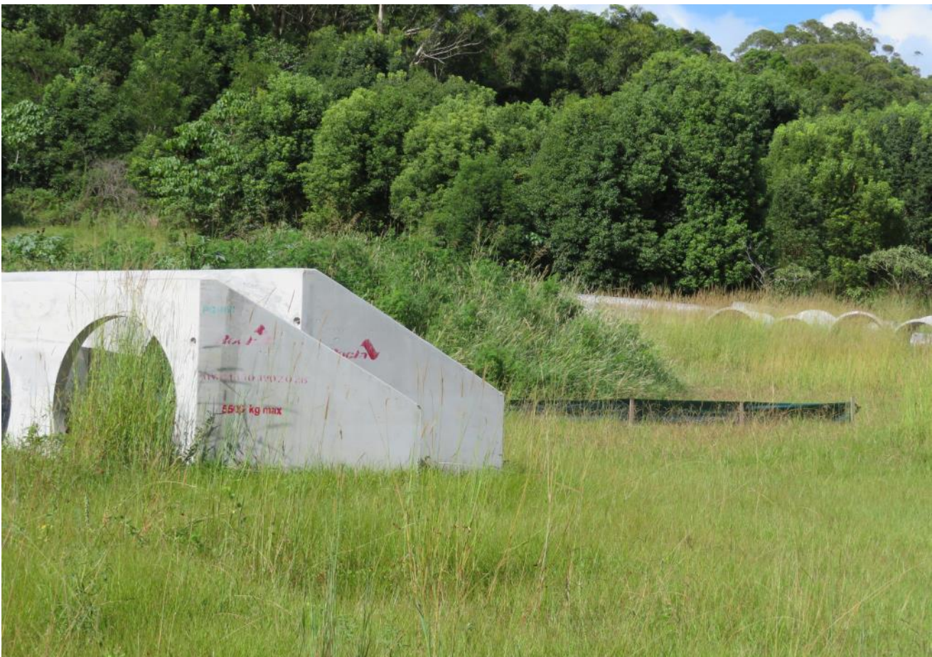
Figure 4 – Photo of vegetated stockpiles and stormwater infrastructure on site ready for installation.
