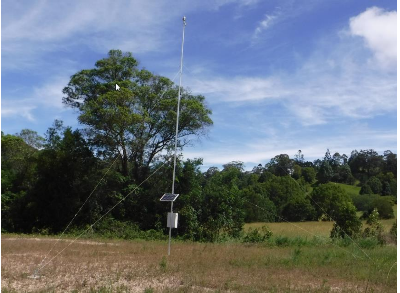
Figure 2 – New meteorological station replaced following the March 30 flood event.
