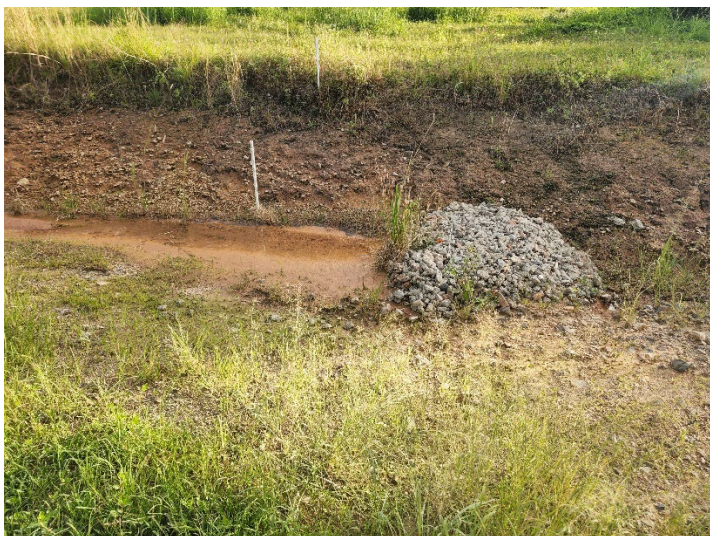
Photograph 5: Haul Road Rock Check ERSED control
