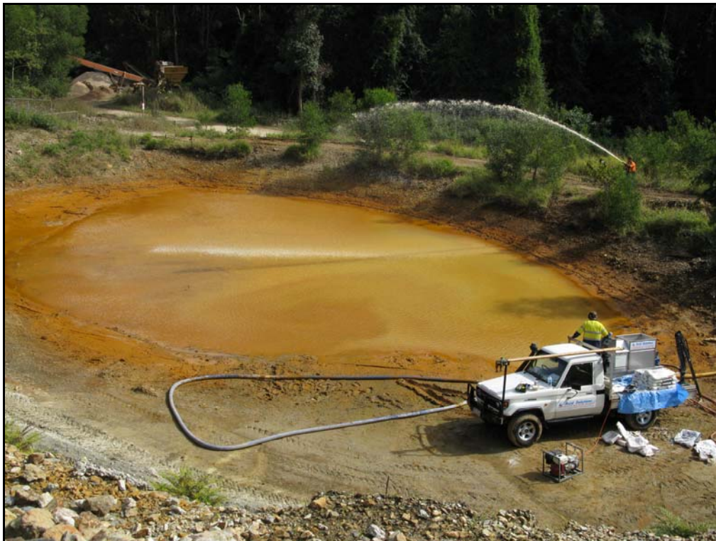
Figure 5: Lime Dosing the Sedimentation Pond in July 2010
