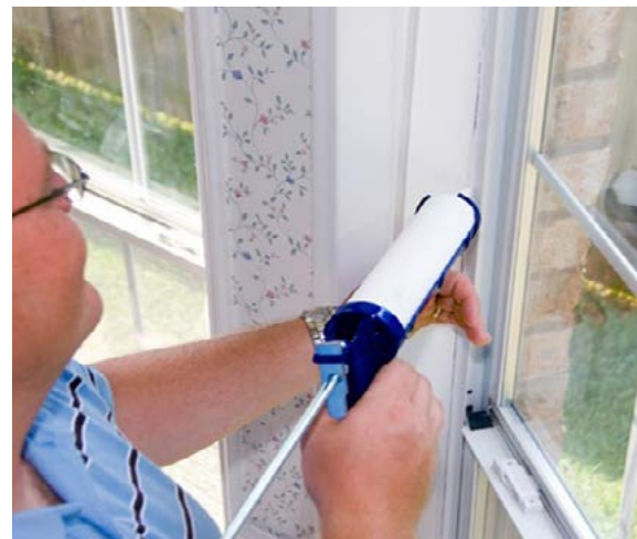
Sealing drafts can make homes more energy efficiency to heat and cool
