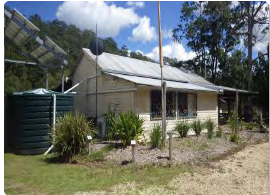
Chillingham Community Centre
