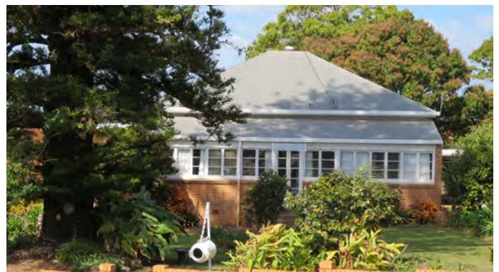
Older dwellings such as this Cudgen farm house add significantly to the locality's built form character.
