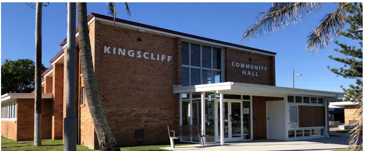
The Kingscliff Community Hall was renovated in 2018.
