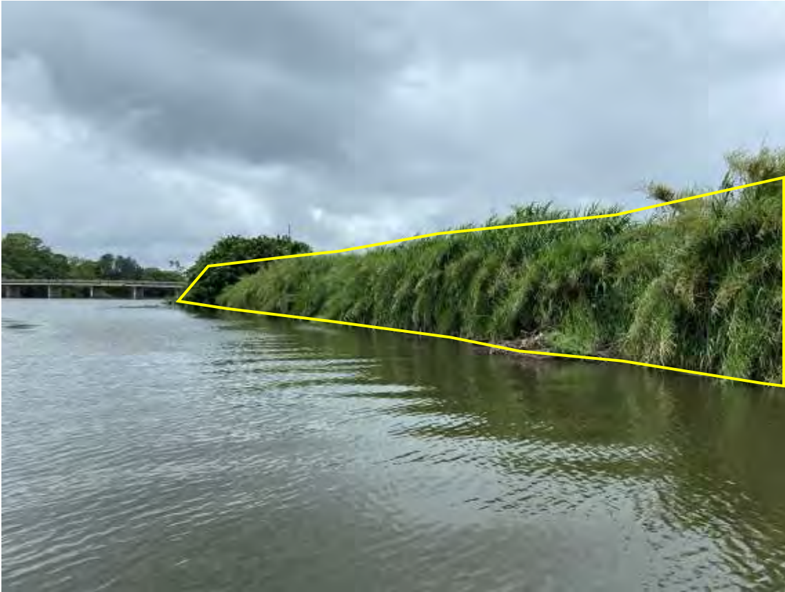
Plate 4: Disturbance footprint looking south along western bank (yellow polygon indicates disturbance footprint)
