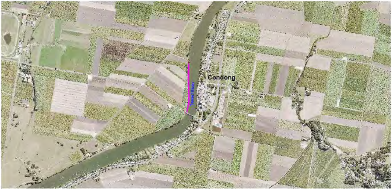
Figure 1: Aerial photograph showing subject site (pink line)
