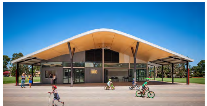
Multi-purpose community facilities within the town centre or Turnock St Precinct. Image: Greenway Architects
