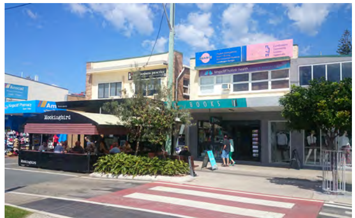
Narrow fronted (fine grain) shops and lower building forms combined with wider footpaths and outdoor dining areas underpin the Marine Parade streetscape.
