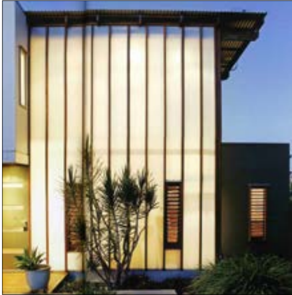
Building forms can be designed to change expression from day to night.
