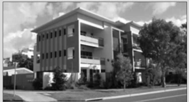
This building has added another half level making the building appear as nearly four levels.
