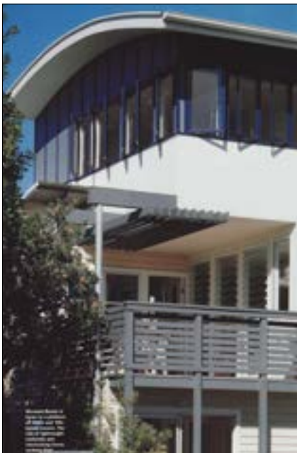
This building has a varied facade with projecting and receding areas, extended by pergolas and stepped with recessed balconies.
