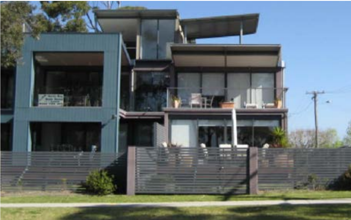
This building appears as two storeys although it is three. The third level is concealed in the roof. Fly roofs taper the building towards the sky reducing the apparent building height.
