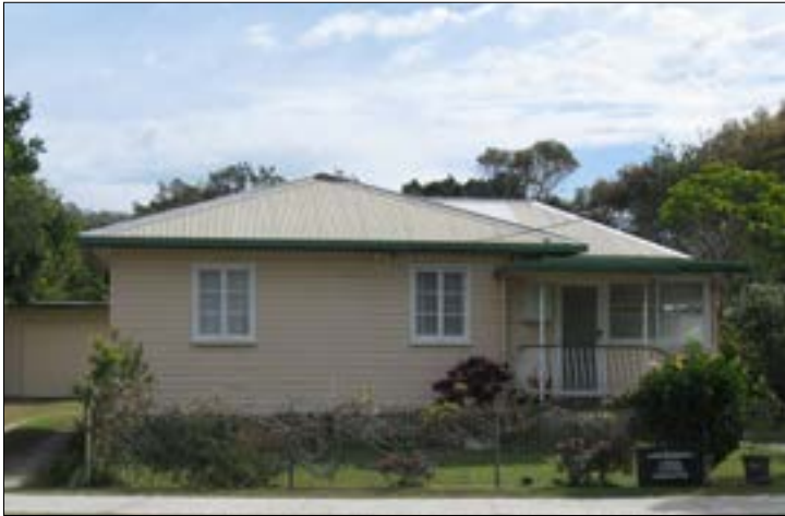
Existing house - lightweight materials
