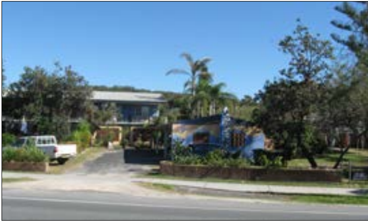
Existing 2 storey flat building
