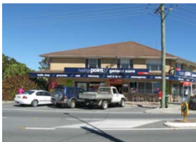
Existing retail building
